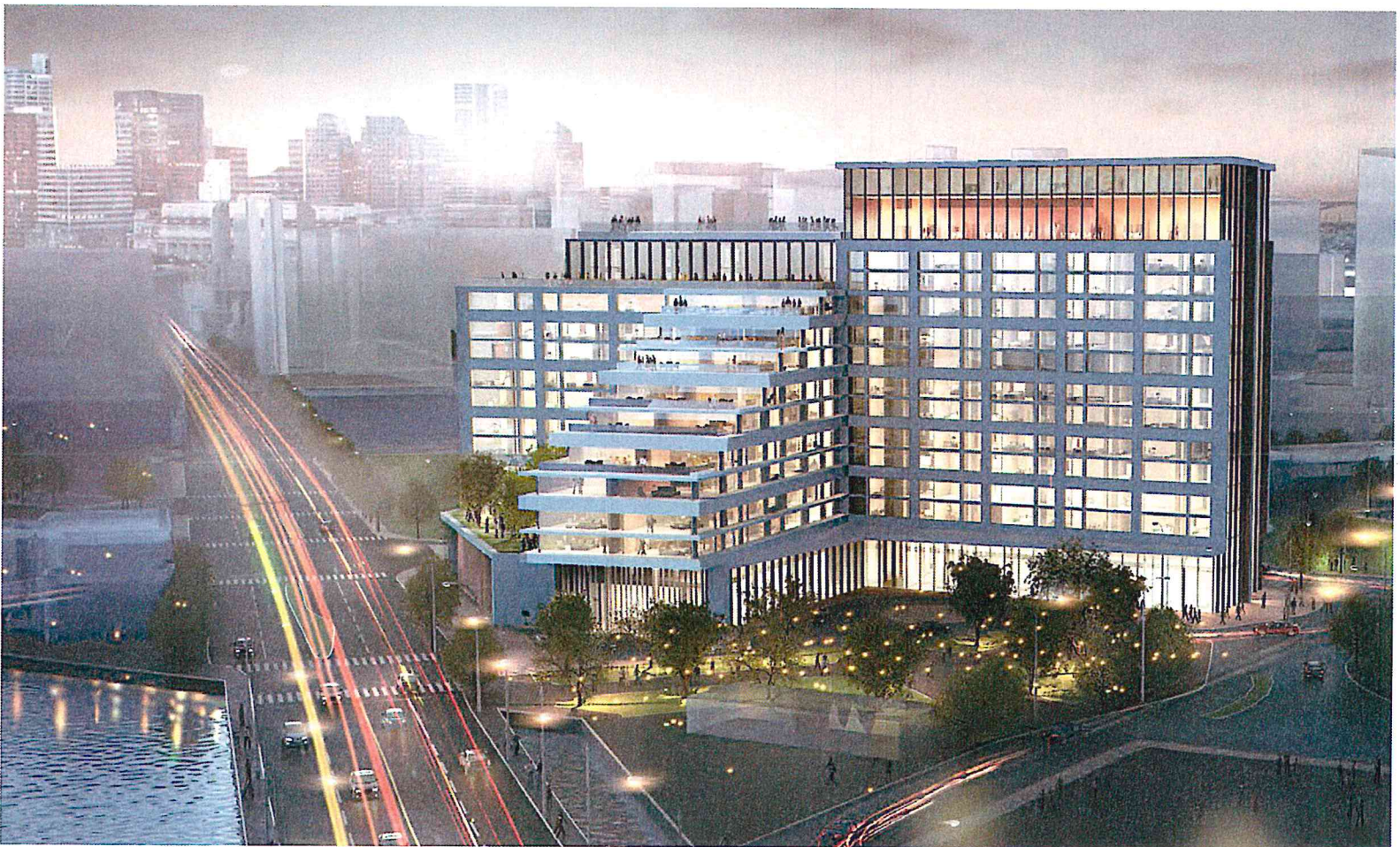
_ENLARGED AERIAL NORTHWEST VIEW
