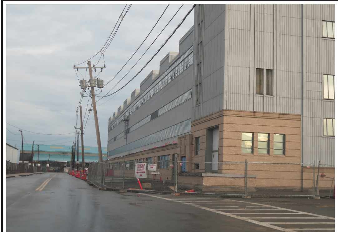
25 Fid Kennedy Blvd (Renovation Under Construction)
