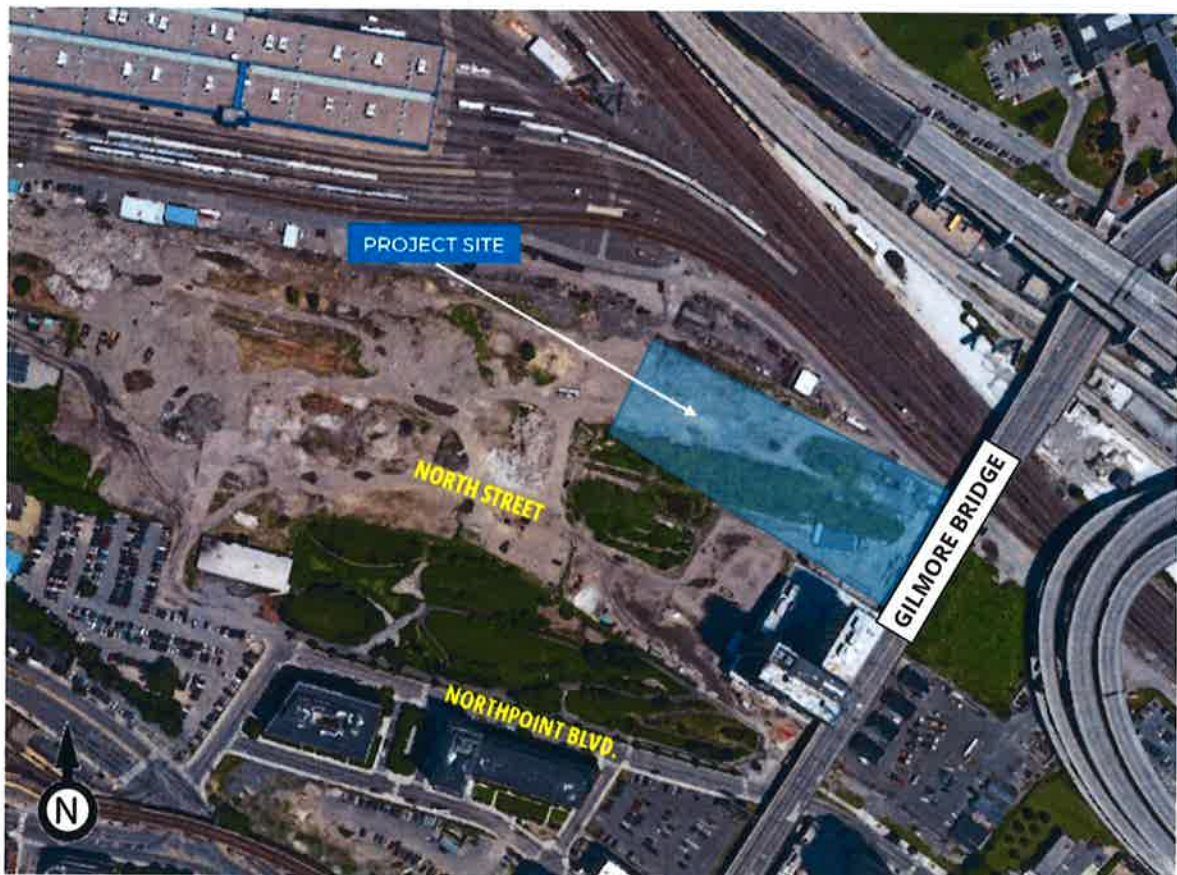
Image 1: Site plan – Aerial view of site and surroundings (courtesy of Google™ Earth)
