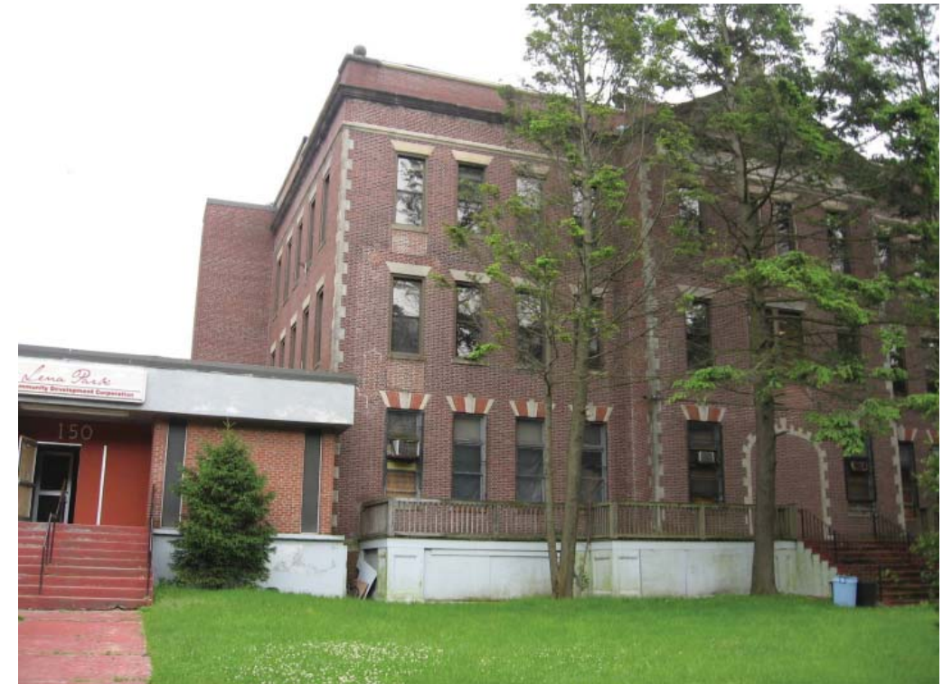
Picture 2: View of northern facade from American Legion Highway.
