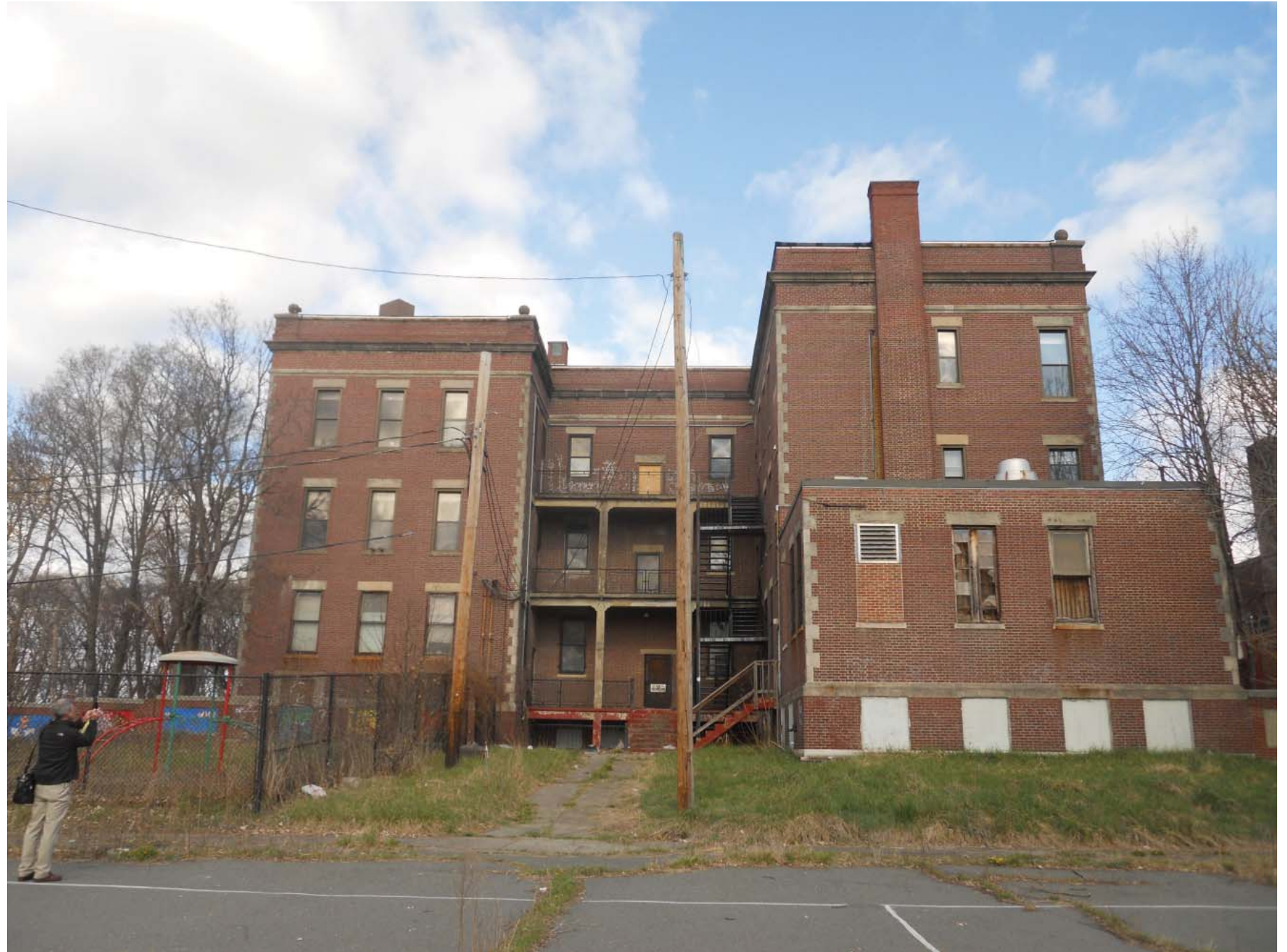
Picture 6: View of southern facade of 1911 building.
