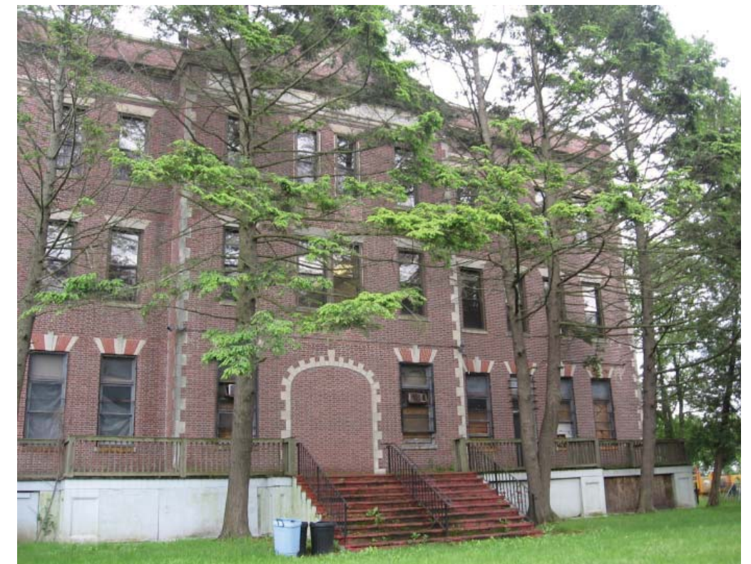
Picture 3: View of northern facade of 1911 building and porch.
