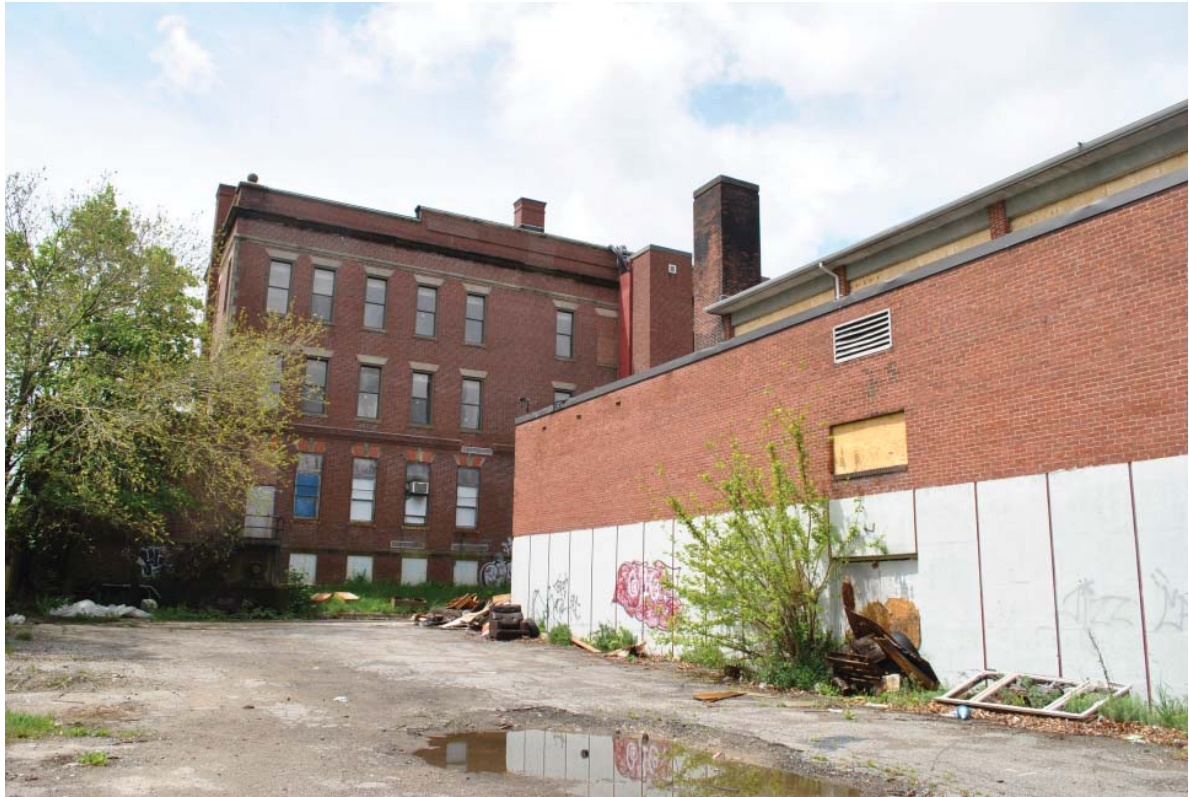
Picture 4: View of 1960 Gymnasium southern facade and eastern facade of 1911 building.
