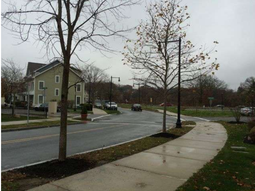
Roadway going through the development
