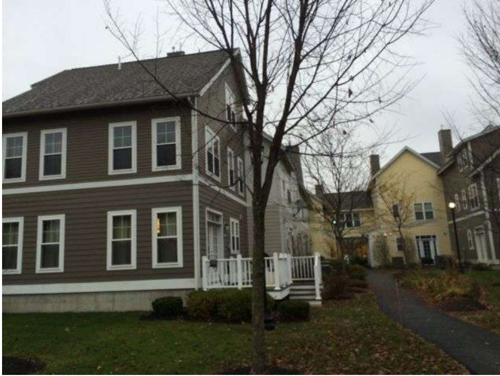
Unit exteriors and walkways
