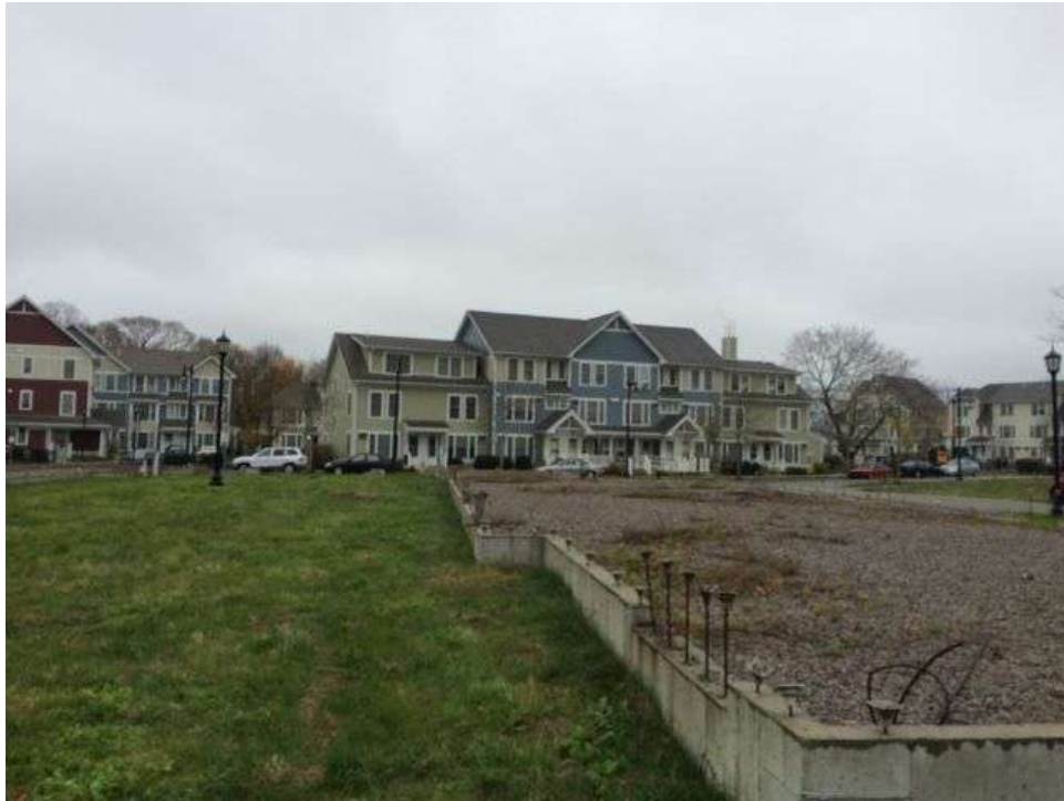
View of condominium townhouse foundations and Phase 1 rental housing
