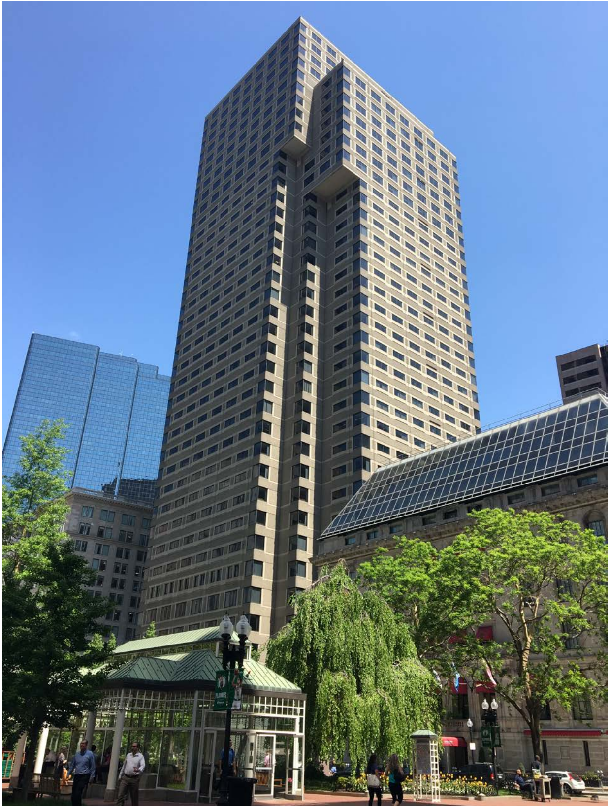
Figure 1-2 Existing One Post Office Square Tower
