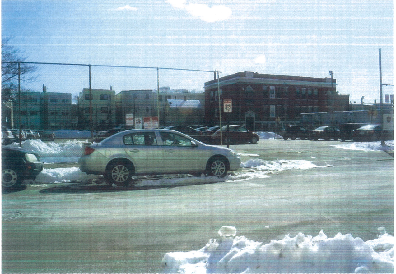
Exterior View of Site
