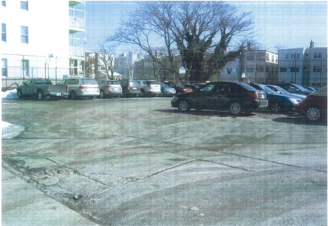
Parking Lot Interior (Looking West)
