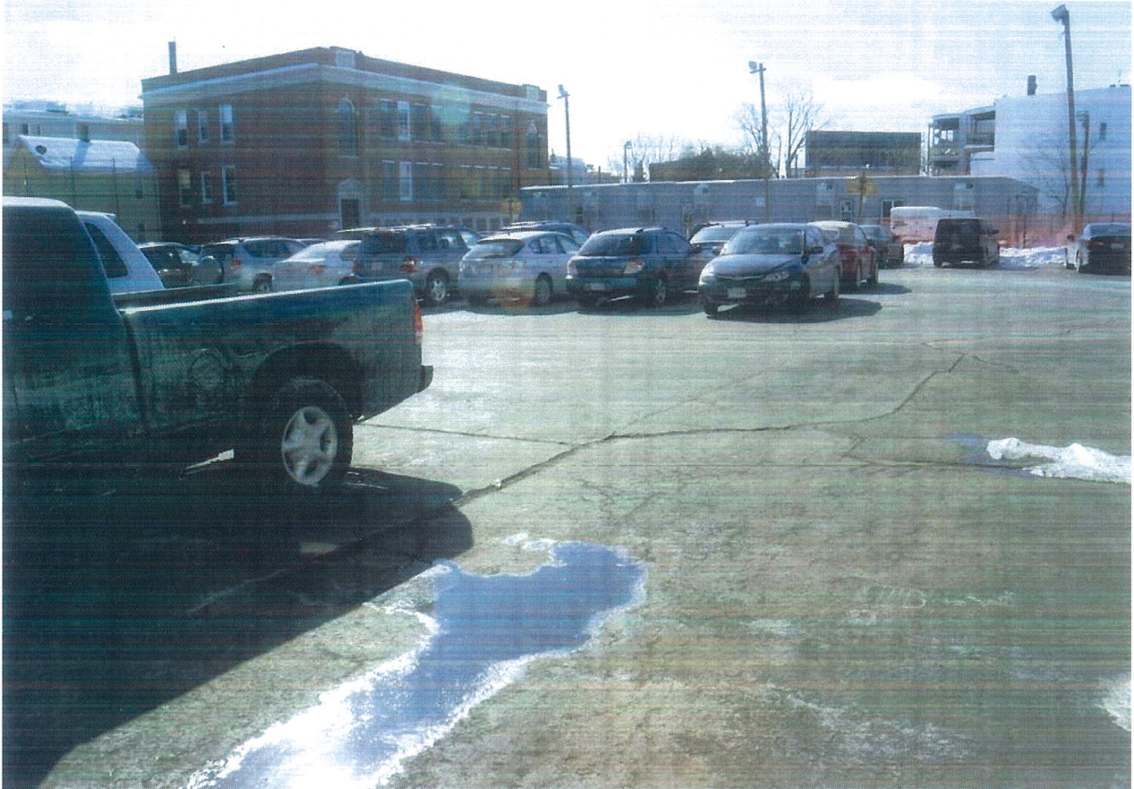
Parking Lot Interior View (Looking East)
