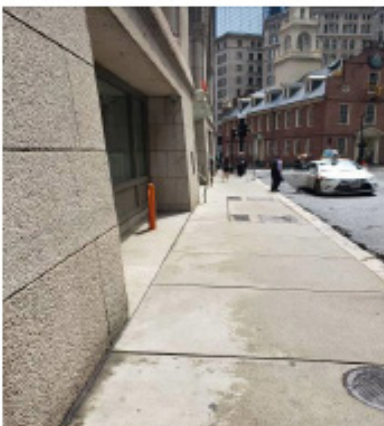
Concrete sidewalk along Court St.
