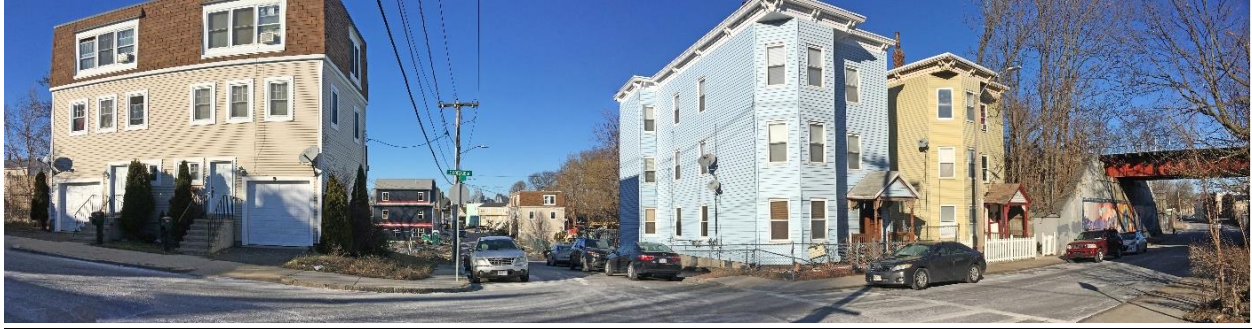
View from E Cottage St. to Robey St.
