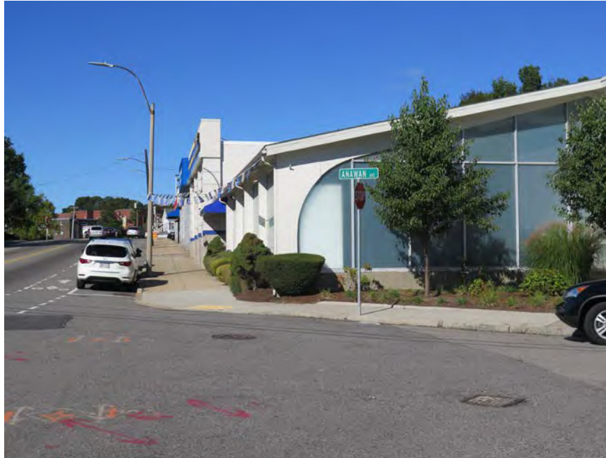
View of Existing Buildings from Anawan Avenue.
