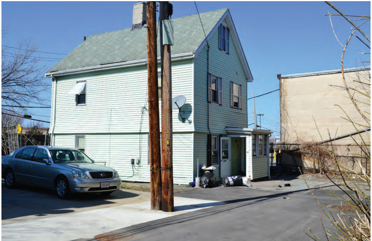
Photograph 6: View of the Site looking east from Baker Court
