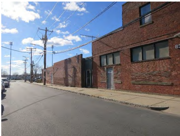
Existing building on site (87-91 Allerton Street) View from east side of Allerton Street facing southerly
