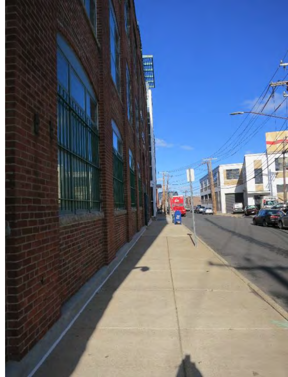
Existing Suffolk Construction headquarters View from Allerton Street facing Northwesterly
