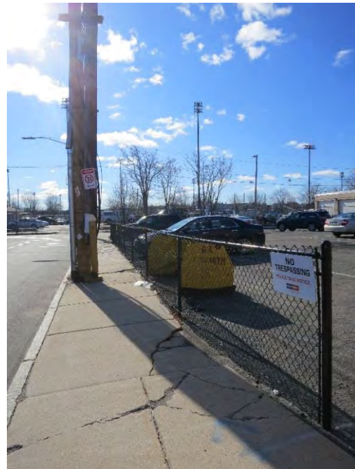
East side of site (Allerton Street) – Near Magazine Street View from Allerton Street facing southerly
