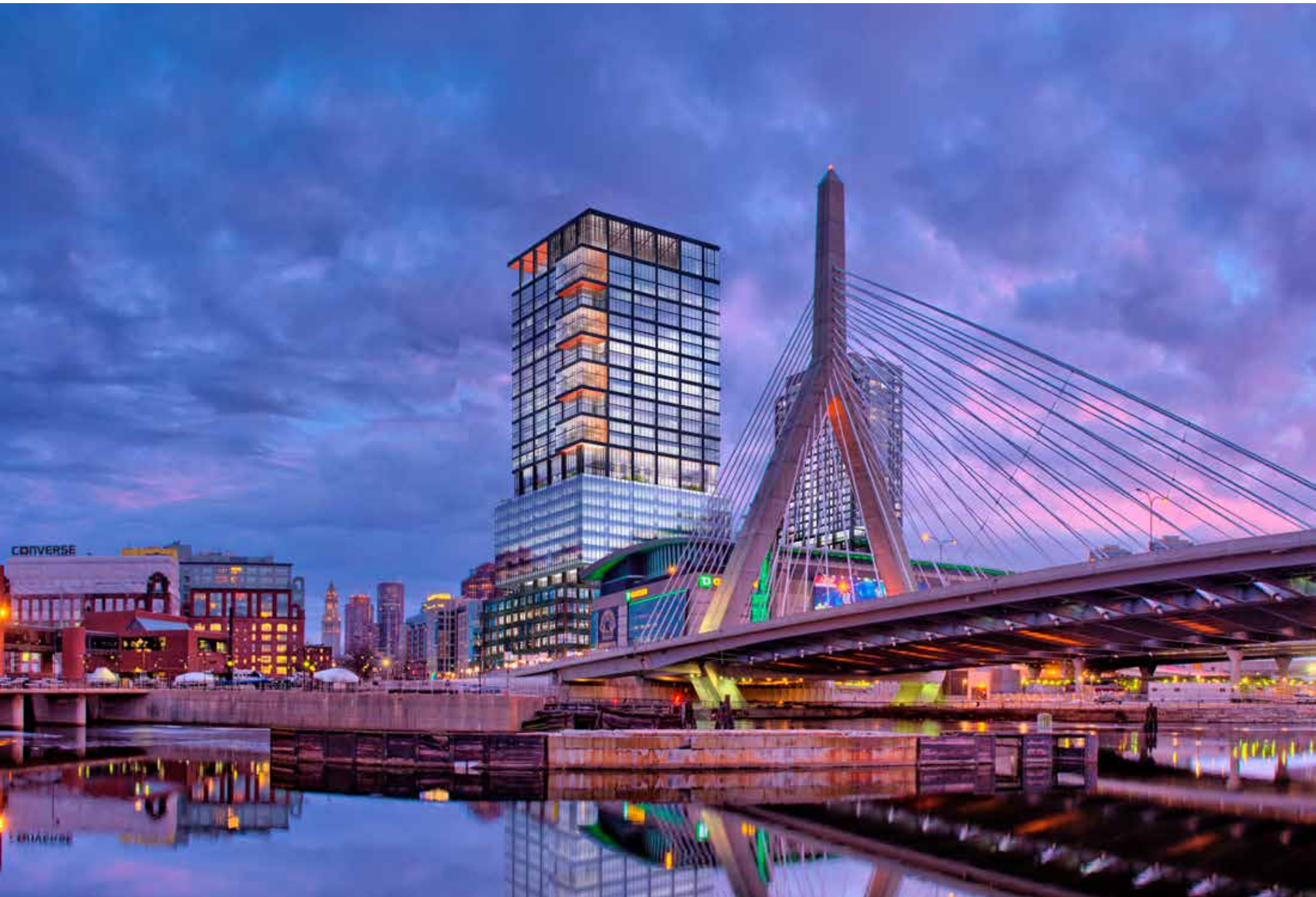
FIGURE 3-3 VIEW FROM NORTH
