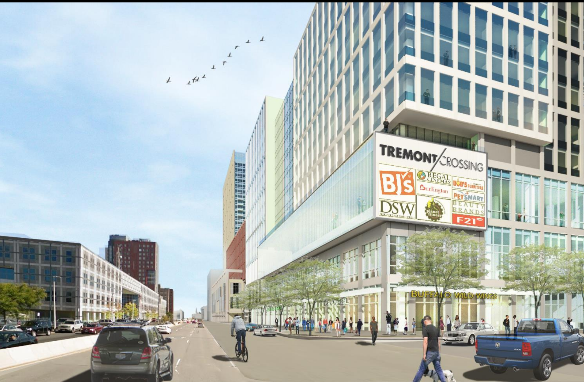
VIEW FROM TREMONT ST. – looking east
