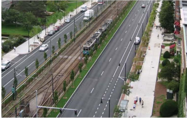
Commonwealth Avenue: Phase 1 improvements
