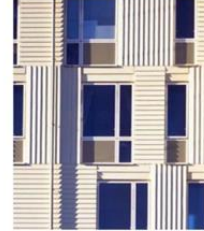
Cast Stone Rainscreen
