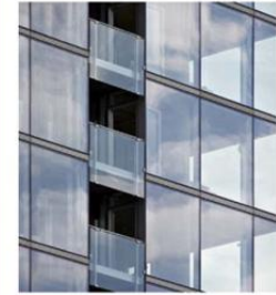
Curtain Wall Glazing
