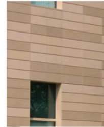
Cast Stone Rainscreen
