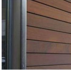
Wood Cladding Rainscreen
