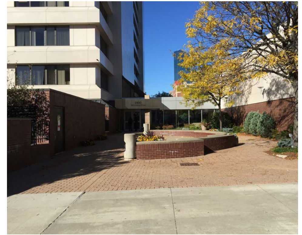
2. Plaza and Existing Lobby Off Harrison Avenue
