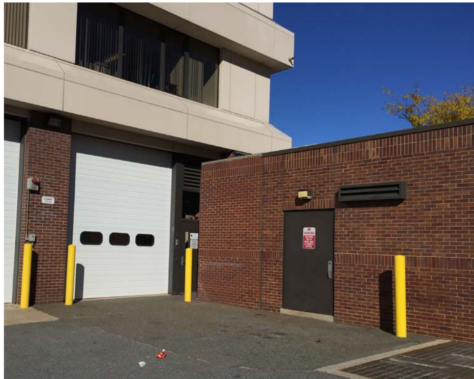
3. Existing Electrical Vault
