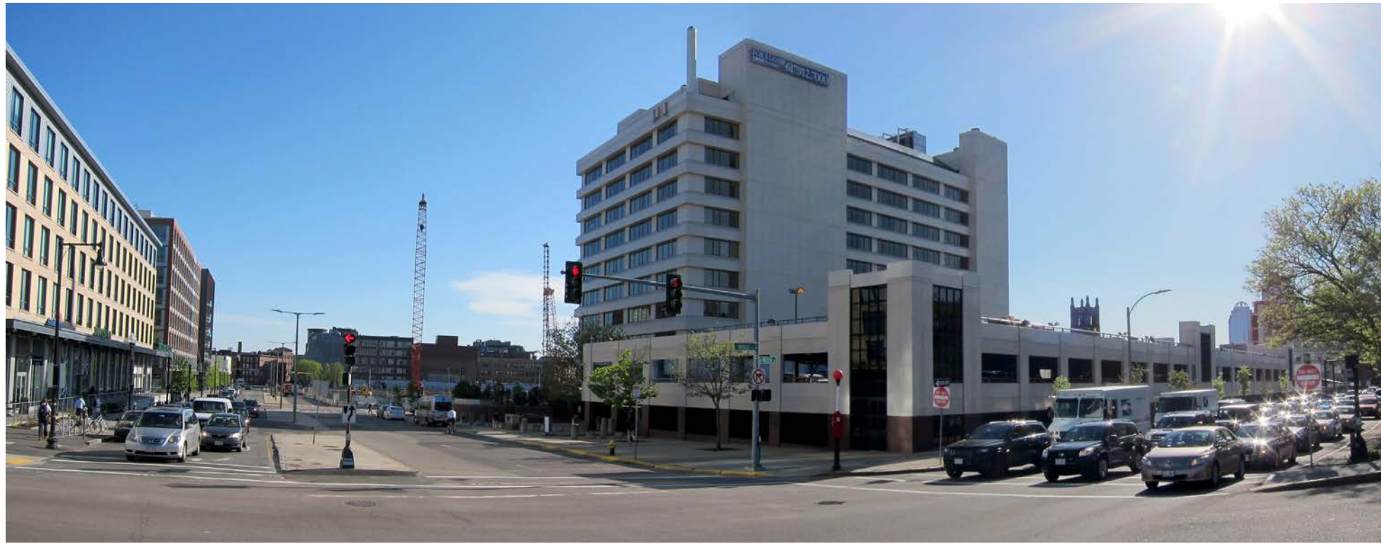
1. View at Corner of Herald Street & Harrison Avenue
