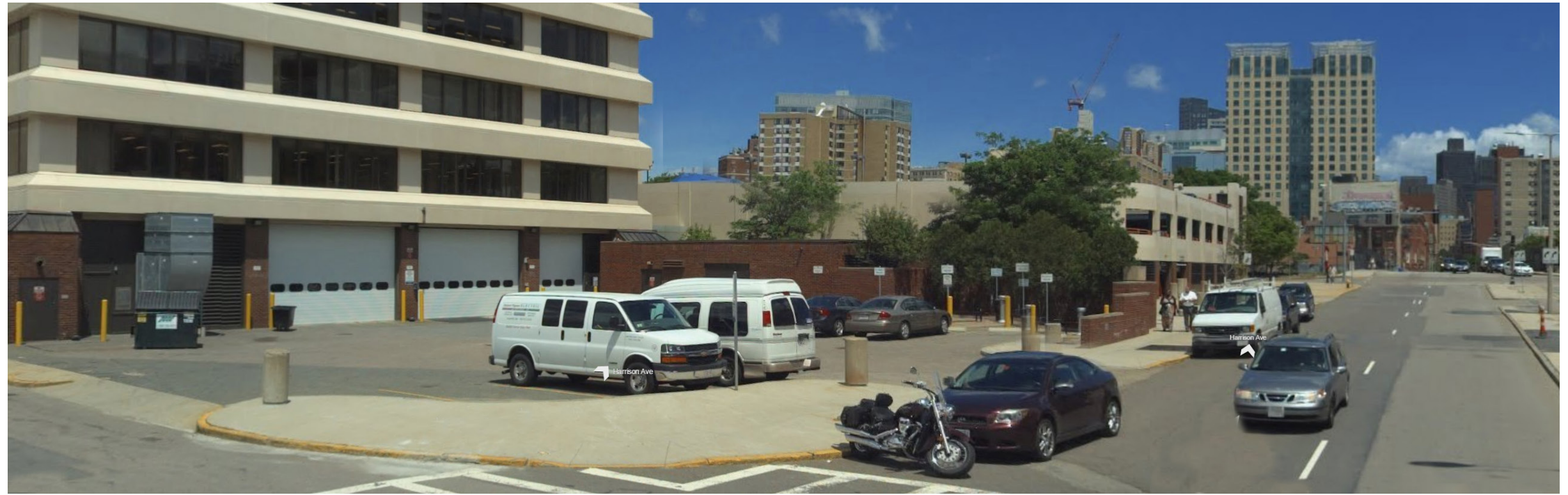
2. Existing Service & Loading Area
