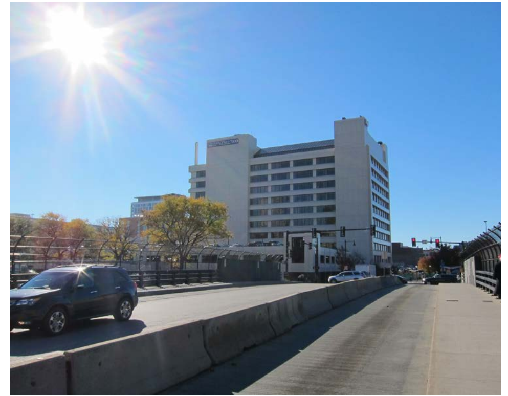
3. View Crossing Washington Street Bridge
