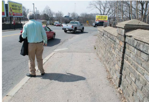
EXISTING SIDEWALK CONDITION
