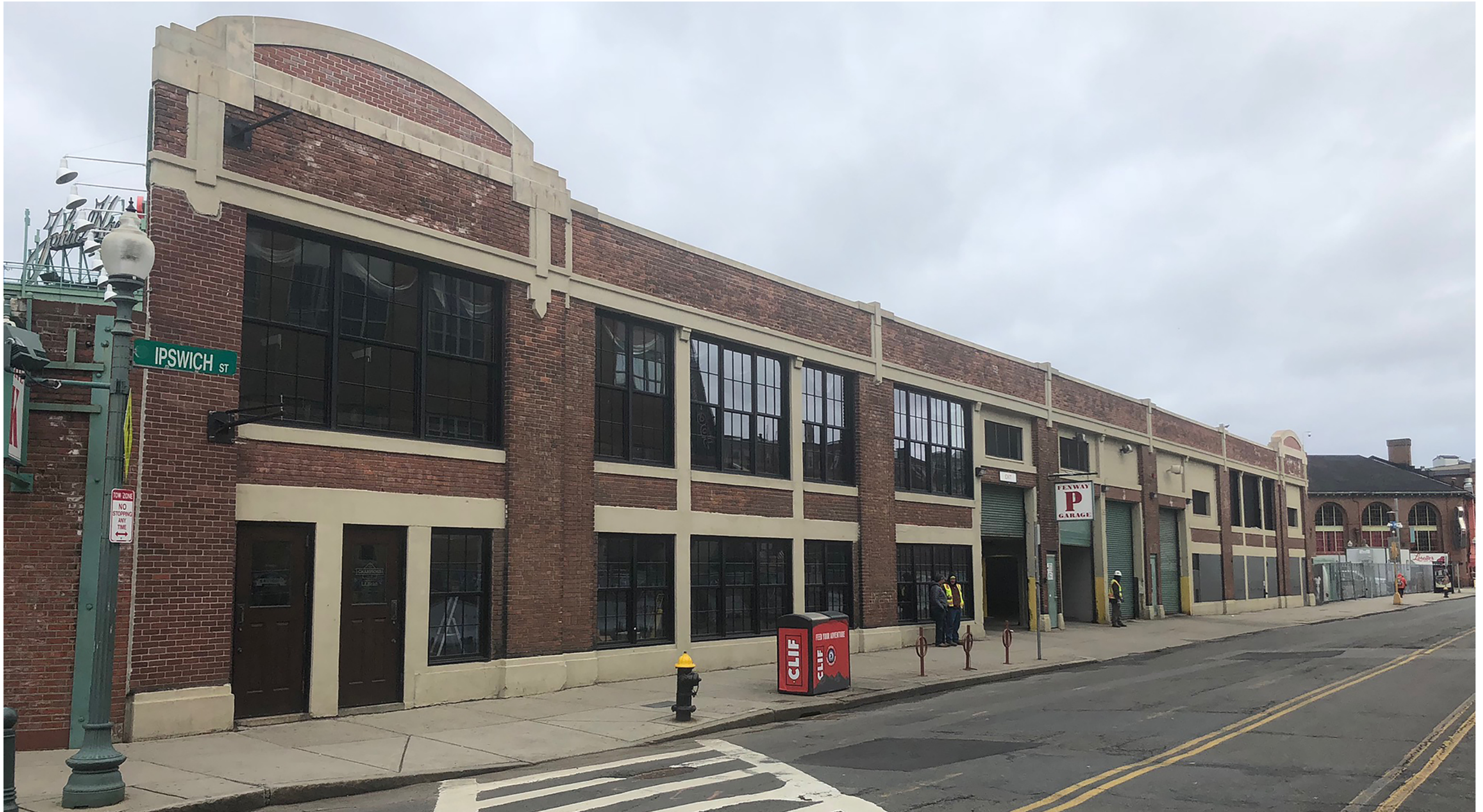
Fenway Garage (Laundry) Building restored windows at Ipswich Street
