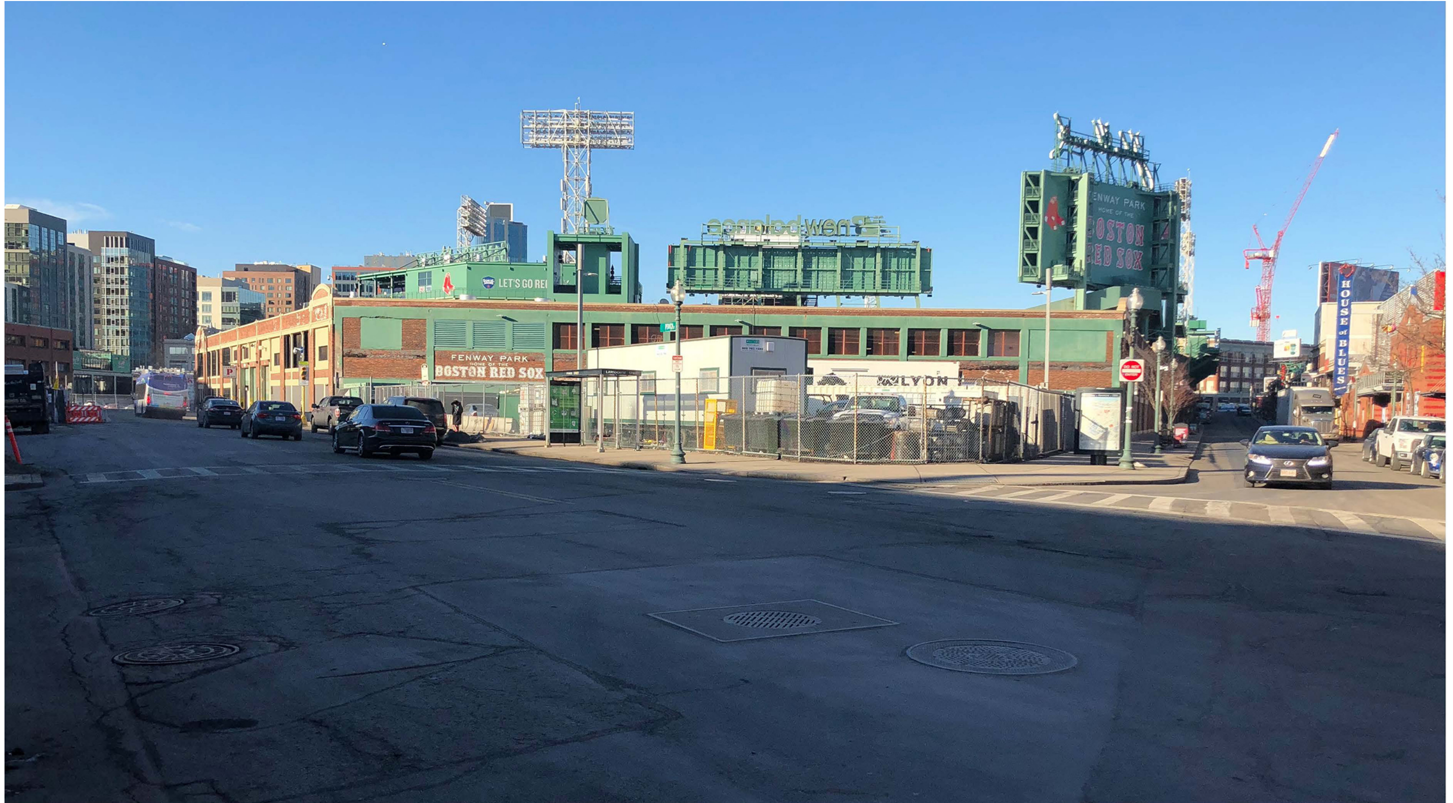
View looking west at intersection of Lansdowne and Ipswich Streets
