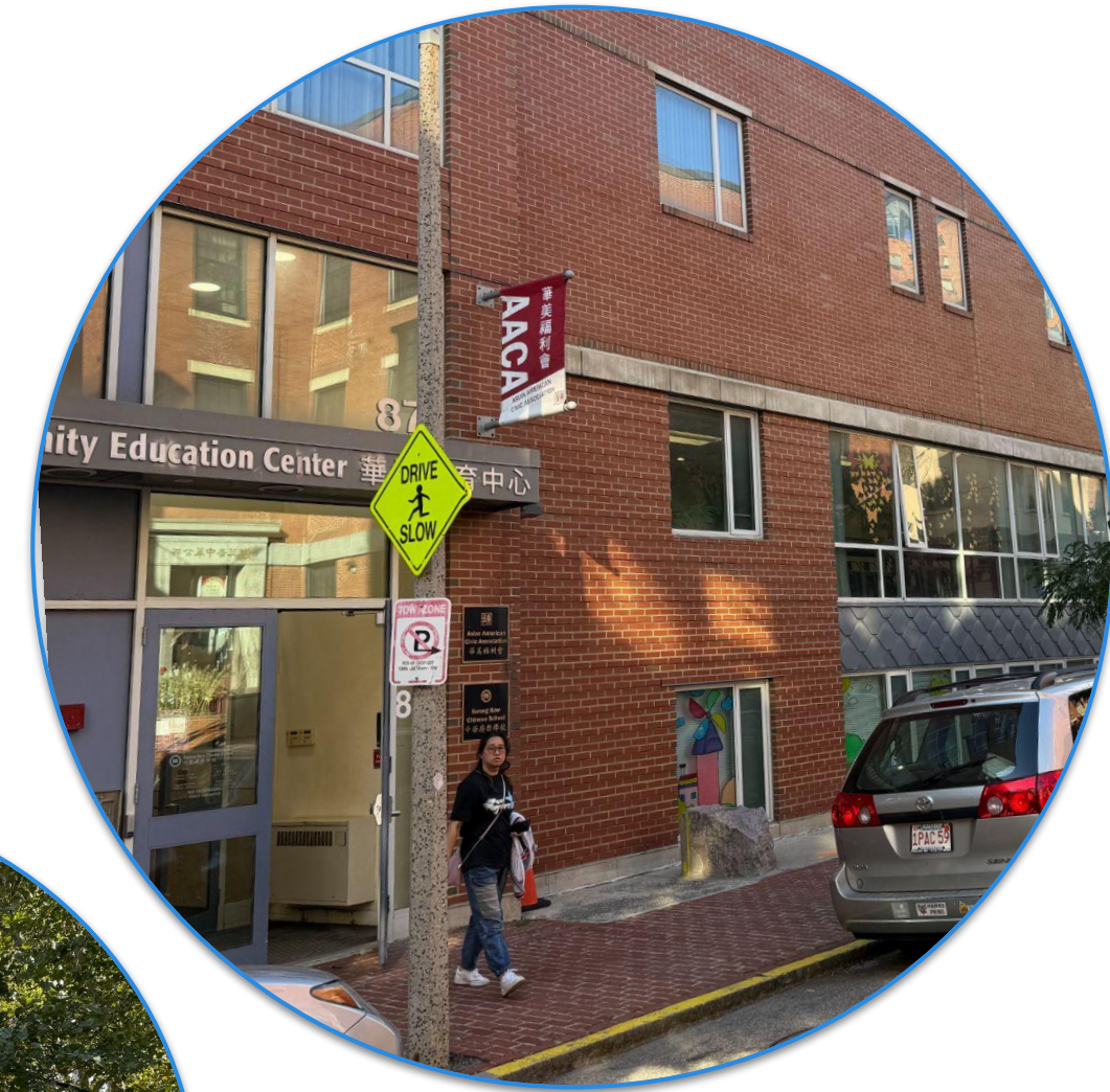
Community uses in institutional buildings
