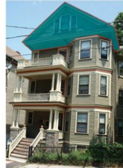
Attic conversion - convert attic into additional unit
