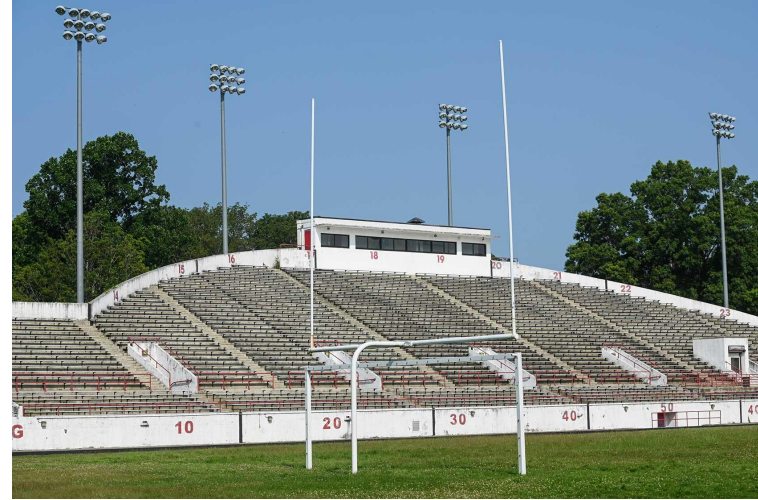
White Stadium, Franklin Park
