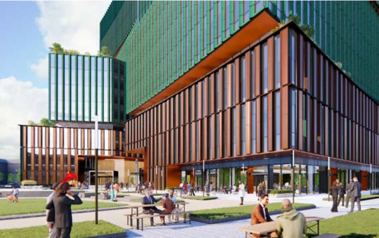
Trees Digitally Removed for Unobstructed View of Façade
