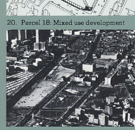
21. Parcel 18 and station site
