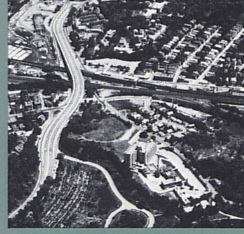
9. Aerial view of station area
