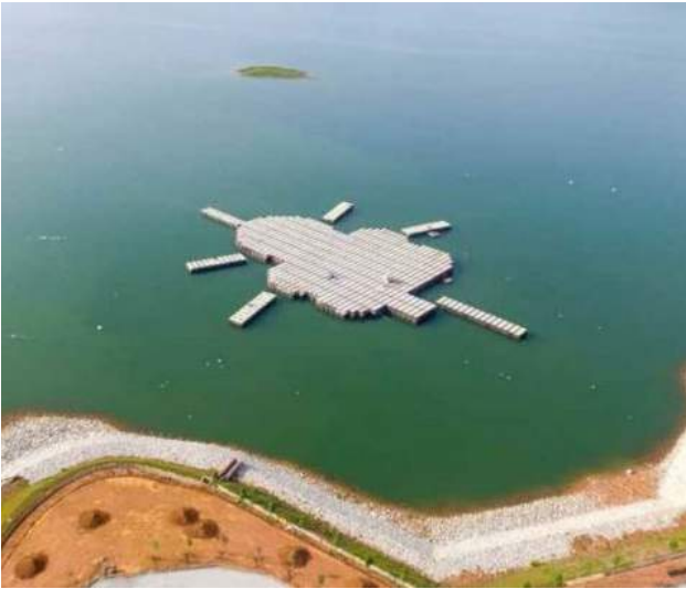
Large floatation base constructed from lots of smaller units
