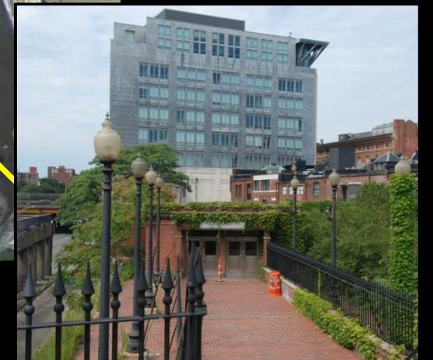
Boylston Street Headhouse
