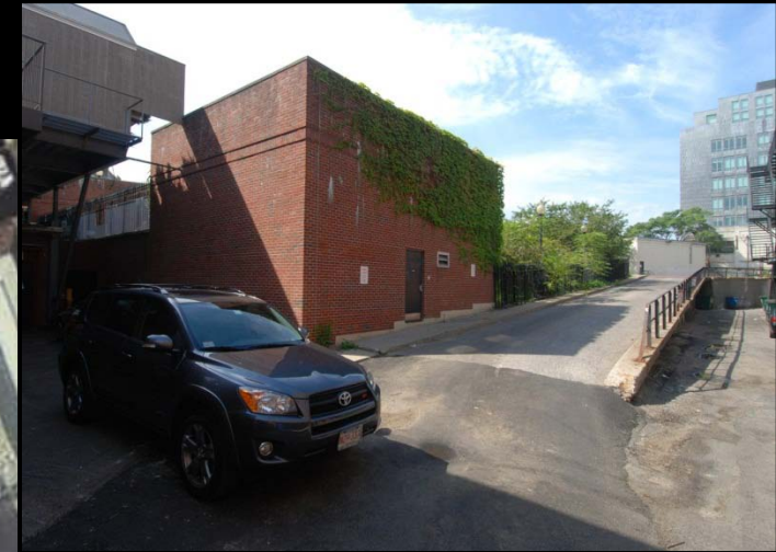
MBTA Ventilation Building
