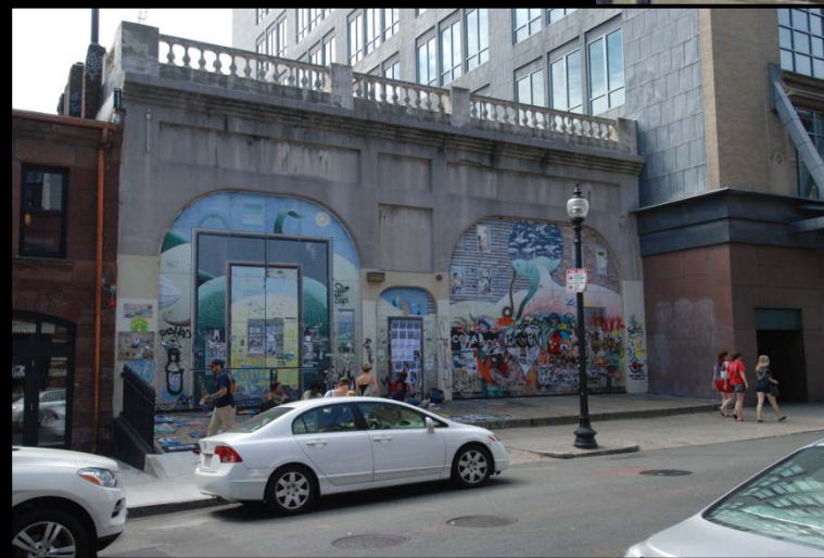
Traction Power Substation
