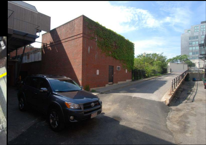
MBTA Ventilation Building
