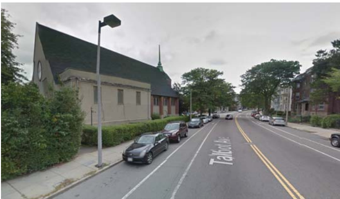
West Elevation at Talbot Avenue
