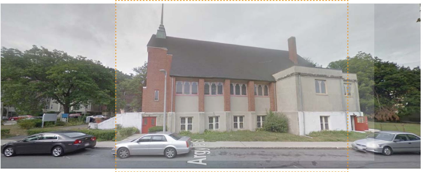
East Elevation at Argyle Street
