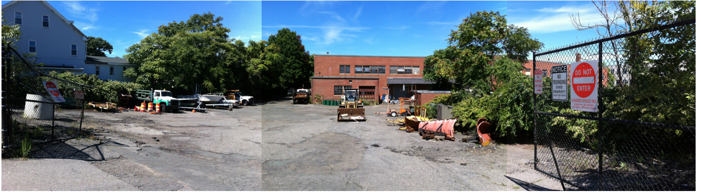
Site, Existing Conditions, View looking northwest from Western Avenue
