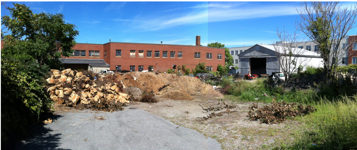
Site, Existing Conditions, View looking northeast from Western Avenue
