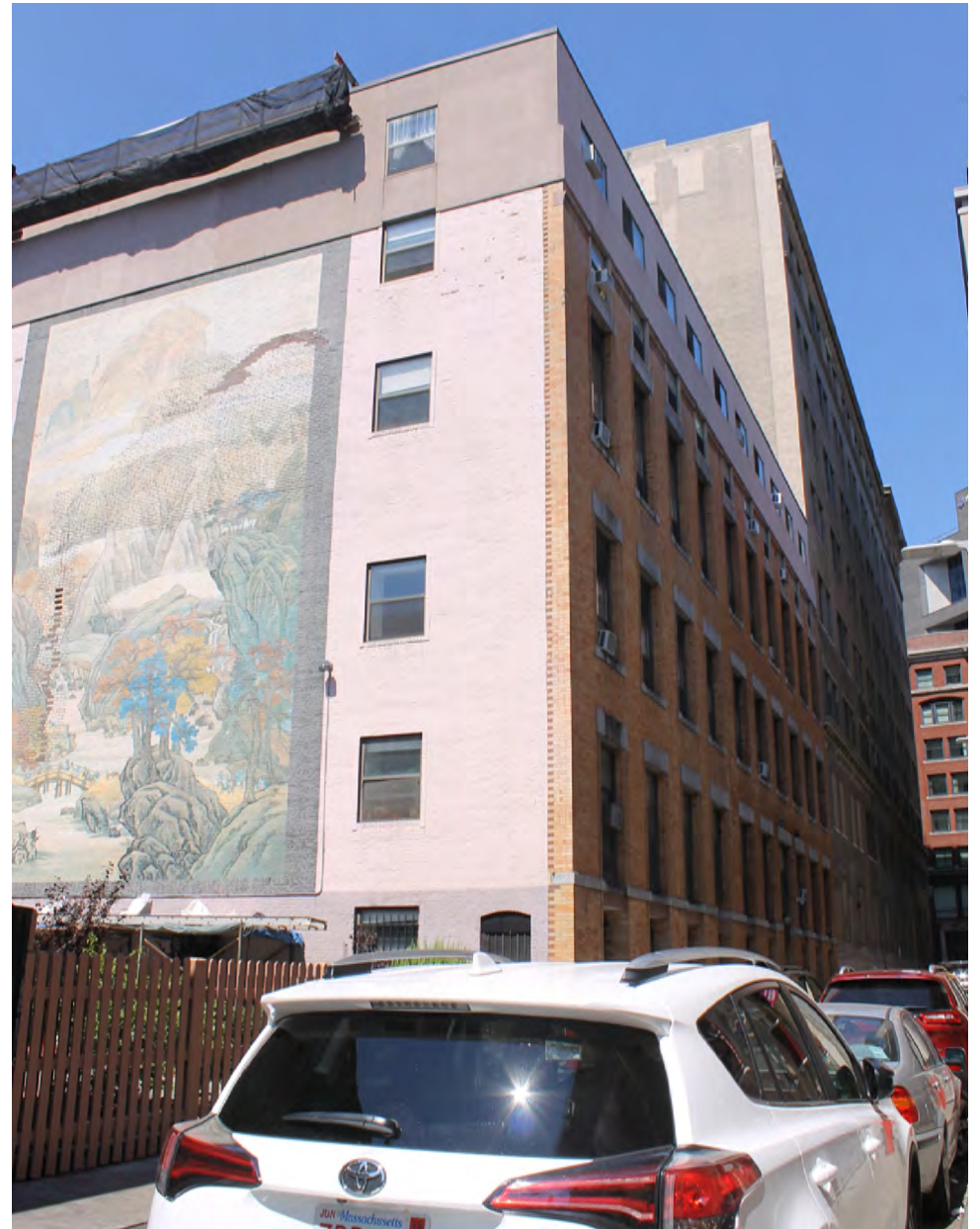
Photograph 4: Rear facade from Oxford Street
