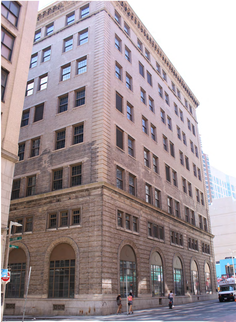
Photograph 3: Essex Street Facade
