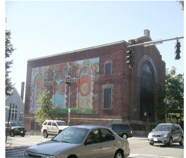
The two story MBTA substation building has been vacant since the 1970's.
