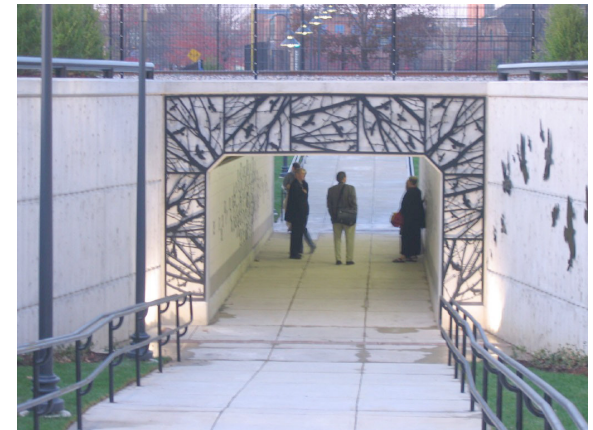
Rehabilitated MBTA underpass in Cambridge, with public art and new lighting.
