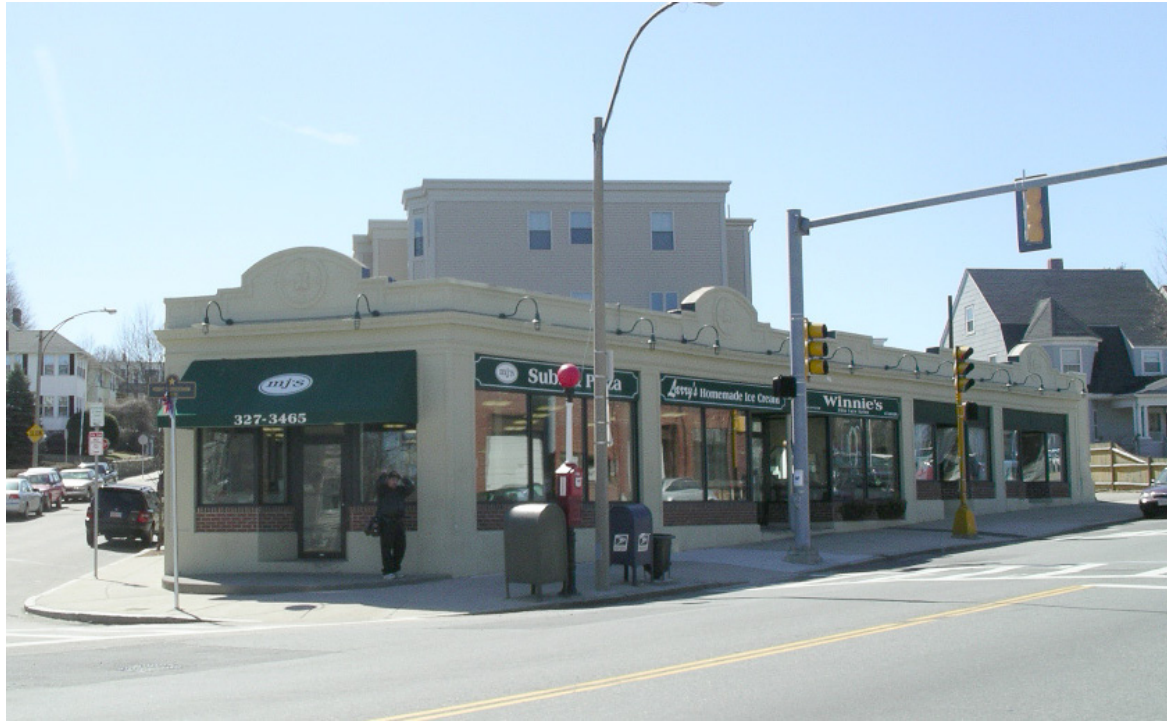
Commercial development throughout most of the neighborhood consists of small stores and service establishments.
