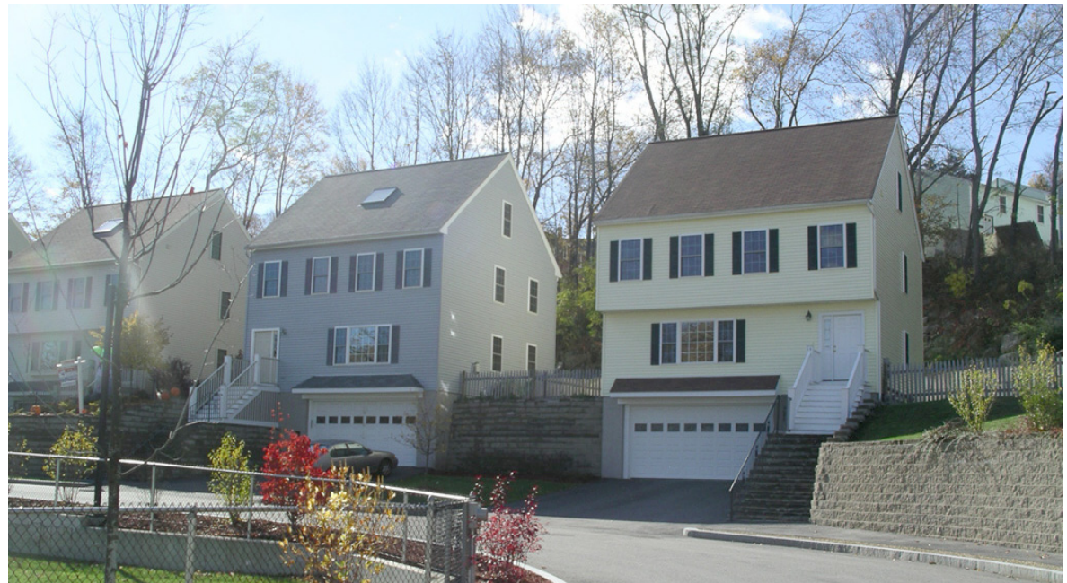
New single family housing on Grew Court.
