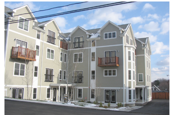
New developments include the Greater Roslindale Medical and Dental Center (top) and residential buildings.
