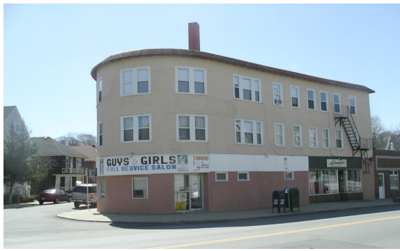
Three-story mixed use buildings provide opportunities for upper level residential use.
