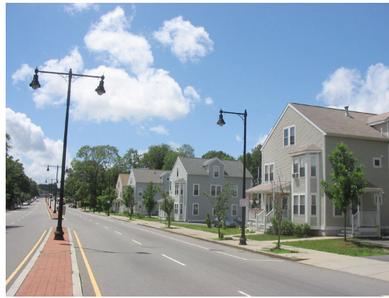
New lighting and median on Hyde Park Avenue.
