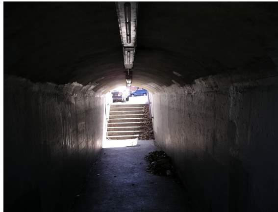
Pedestrian tunnel at the Bellevue Commuter Rail Station.
