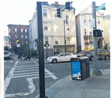
4. Corner of Tremont St. and St. Alphonsus St. - ADA/MAAB compliant pedestrian ramp with truncated dome insert.
