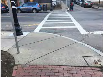
1. The existing pedestrian ramp at the corner of Tremont Street and Worthington Street does not meet ADA/MAAB code and will be replaced with a compliant ramp including truncated domes insert.
