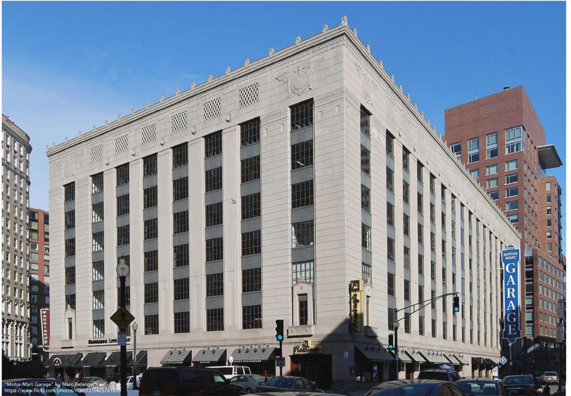
Motor Mart Garage Boston, Massachusetts
