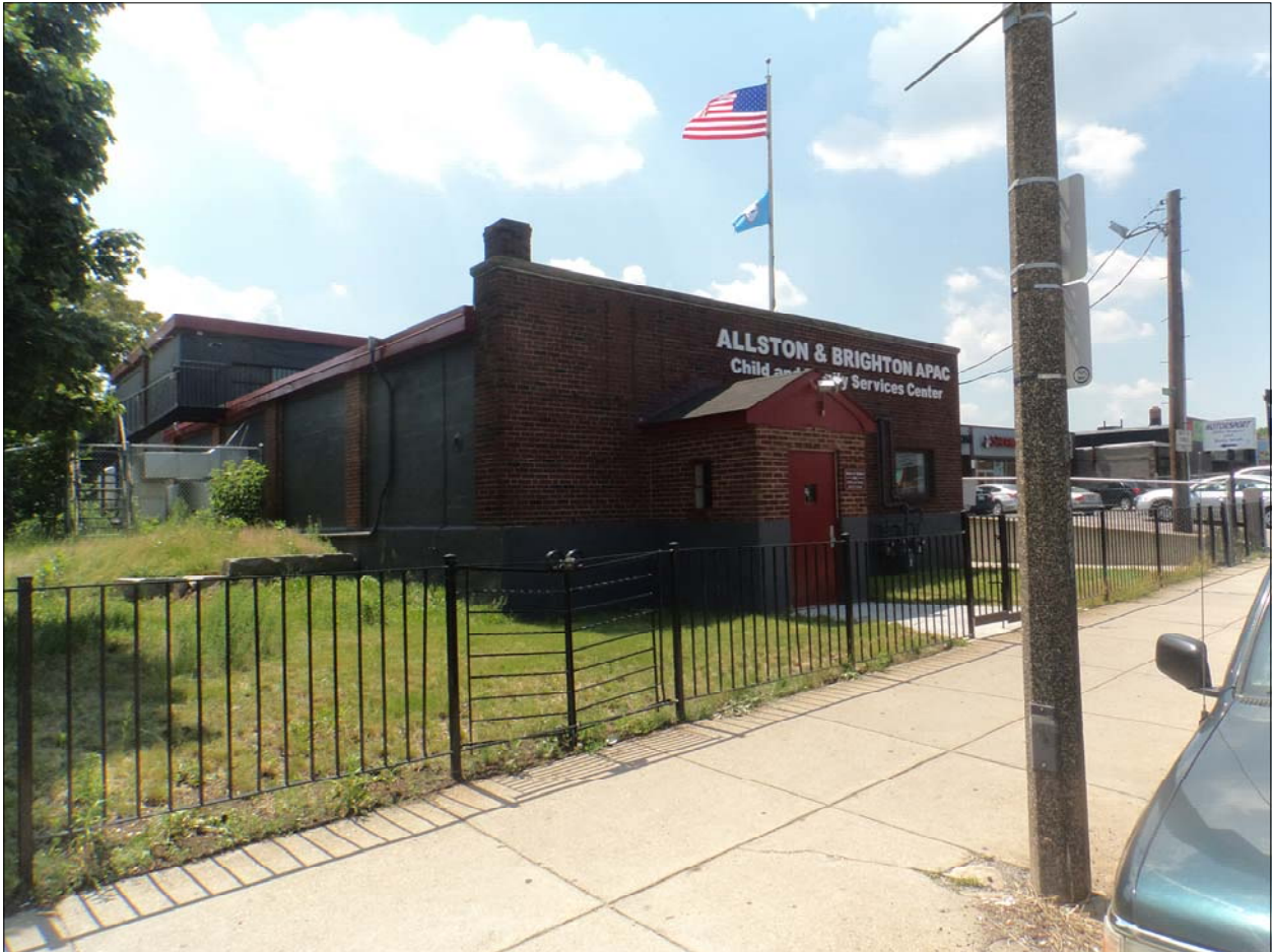
PROJECT SITE ADJACENT BUILDINGS: WEST SIDE
