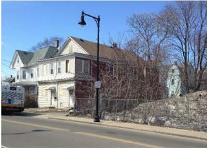
SOUTH-WEST CORNER OF SITE FROM RIVER ST.
