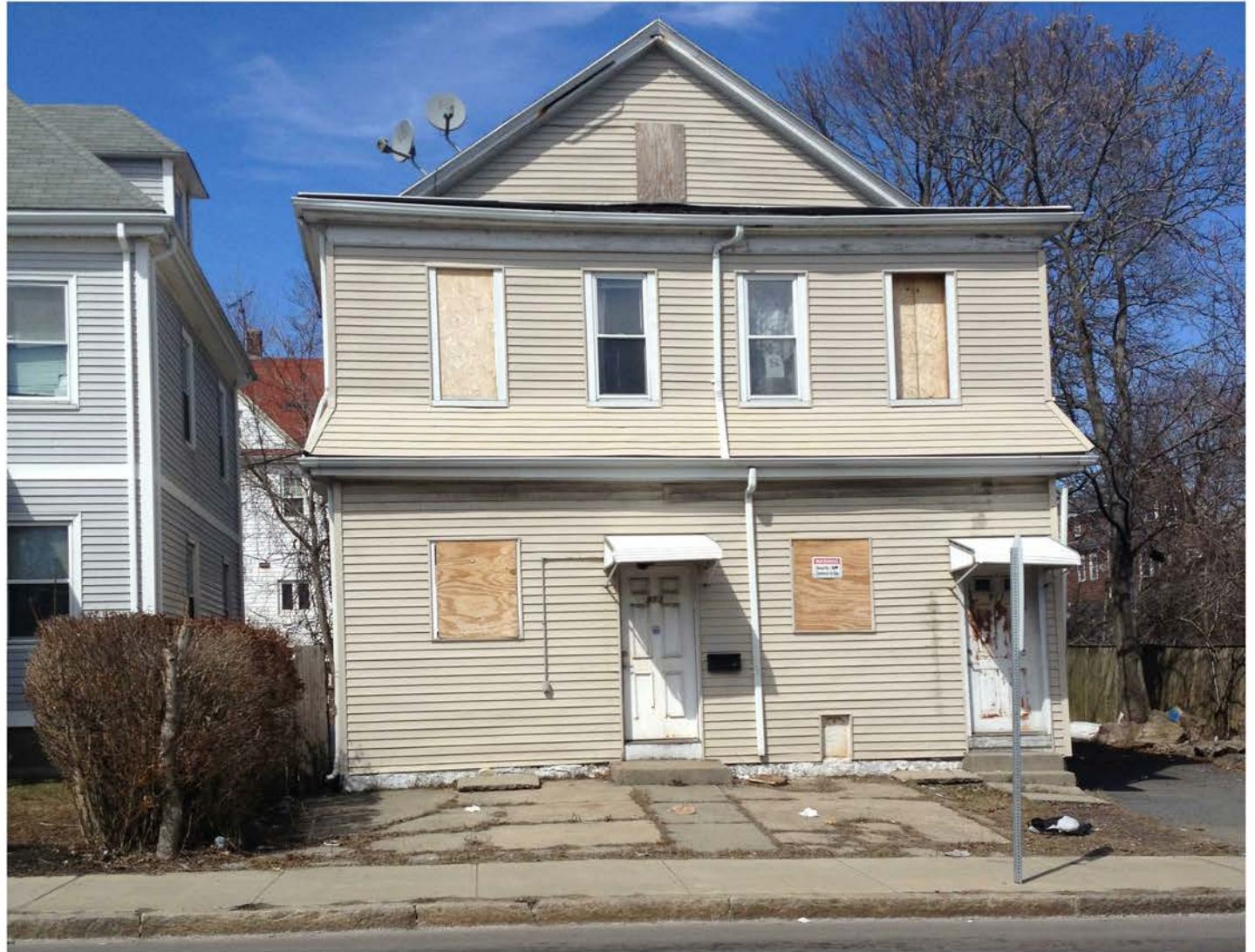
VIEW OF ABANDONED HOUSE ON RIVER ST.
