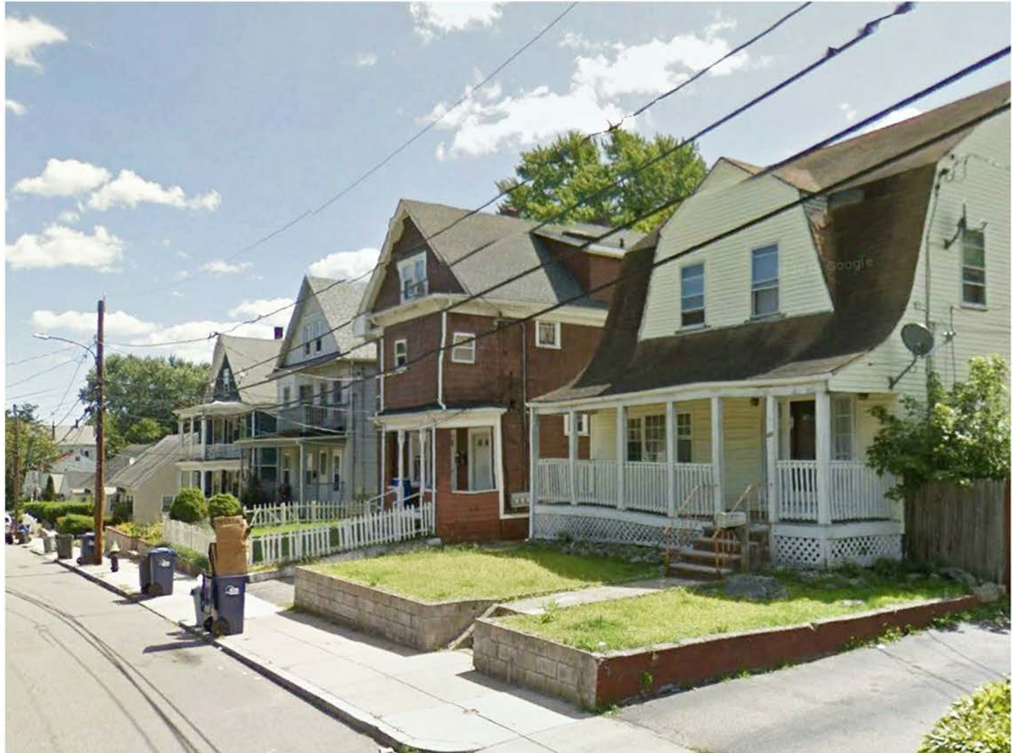
FRAZER ST. RESIDENCES BACKING UP TO NORTH BORDER OF SITE
