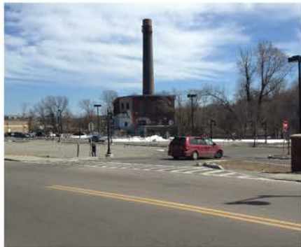
VIEW FROM RIVER ST. LOOKING SOUTH-EAST
