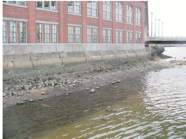
Figure 2-18 Existing Conditions Photos - Building 114 source: Fort Point Associates, Inc.
