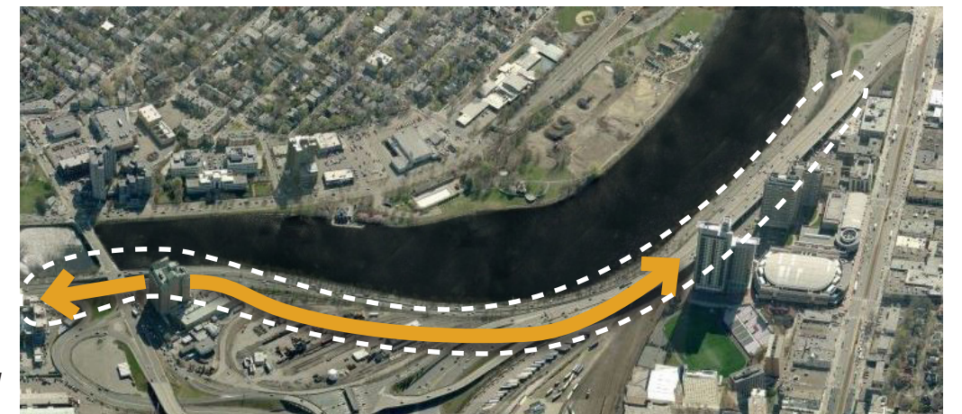
The current alignment of Soldiers Field Road and portions of the MassPike are contained within a narrow corridor along the Charles River.
