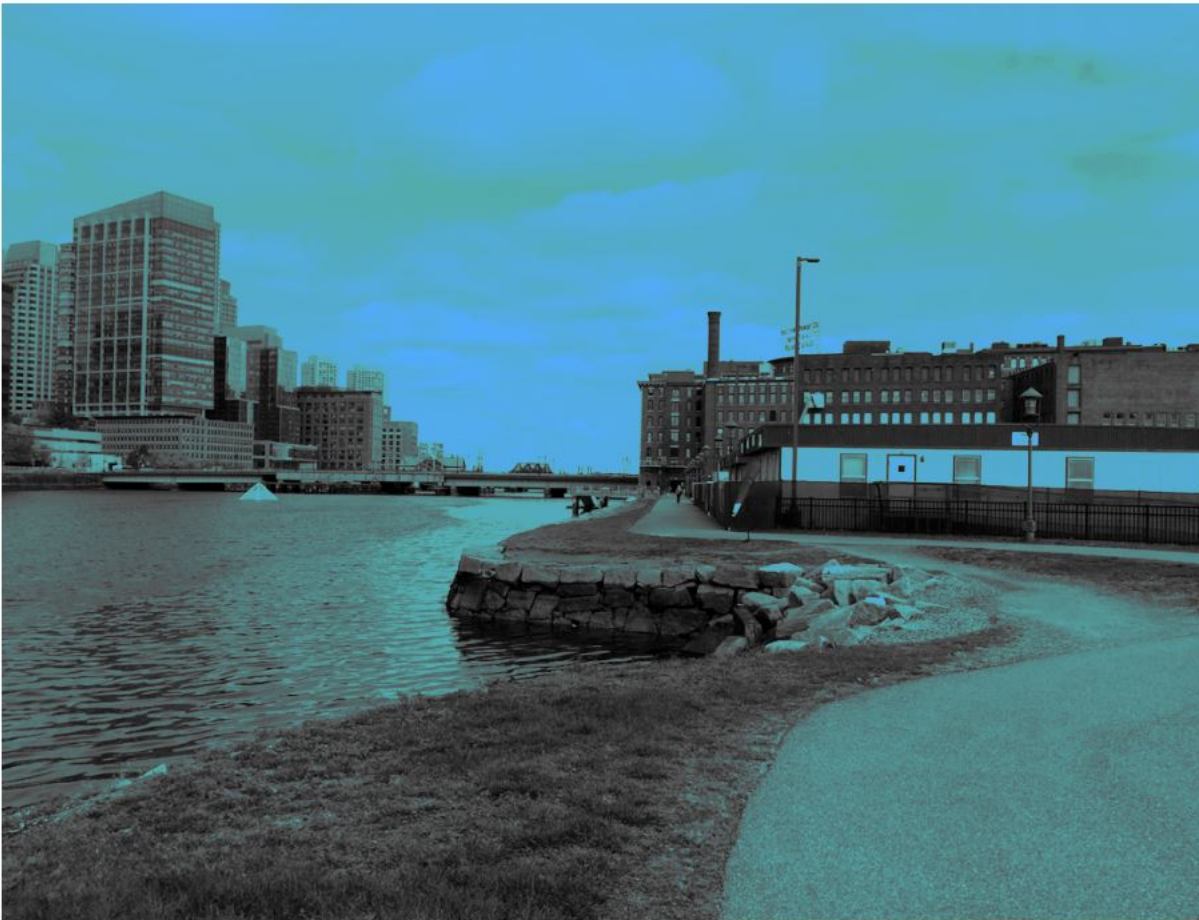
Figure C-4. Coastal bank present at the project site, comprised of both sections of the channel wall and of a gentler, cobble and riprap slope (Coastal Resilience Solutions for South Boston 2018).
