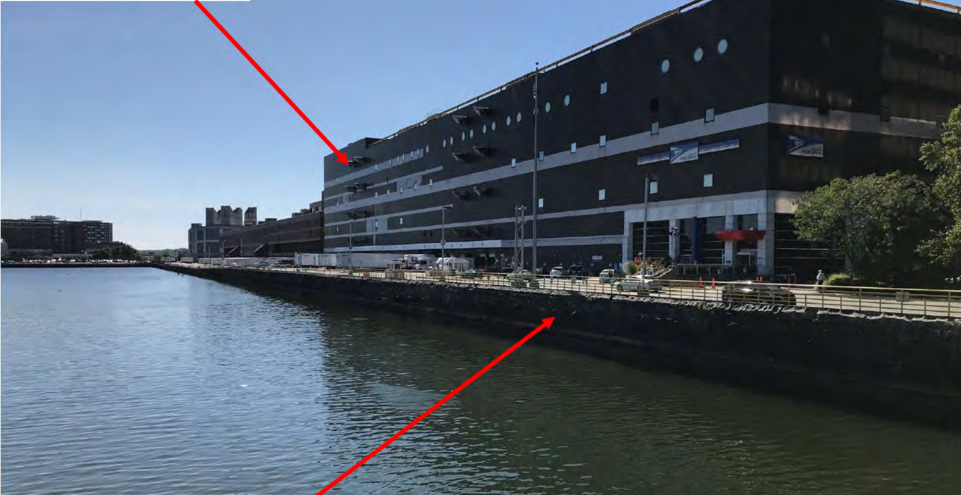
West Side of Fort Point Channel Seawalls
