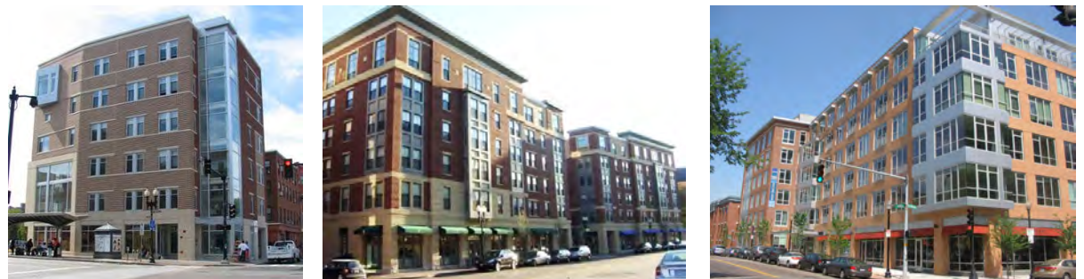
The stepbacks, window and corner details, and cornice lines help to articulate these buildings.
