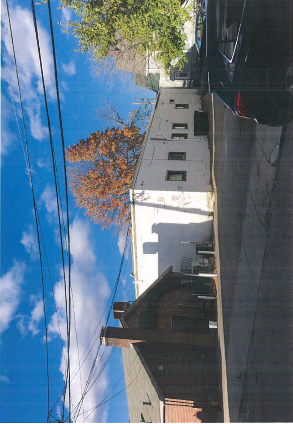
214 Market Street – Rear View
