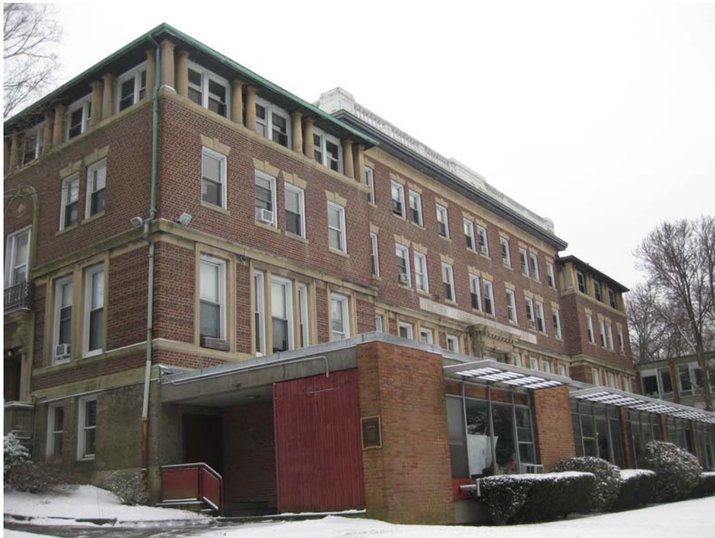
8. 1914 Building and 1950s addition (west elevation)
