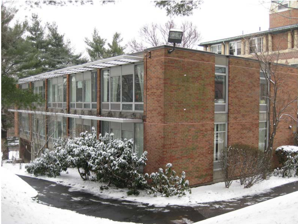
5. 1950s addition to south pavilion (south and east elevations)
