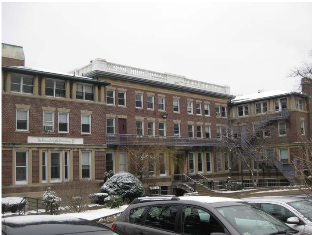
2. Home for Little Wanderers, 1914 Building (east elevation)
