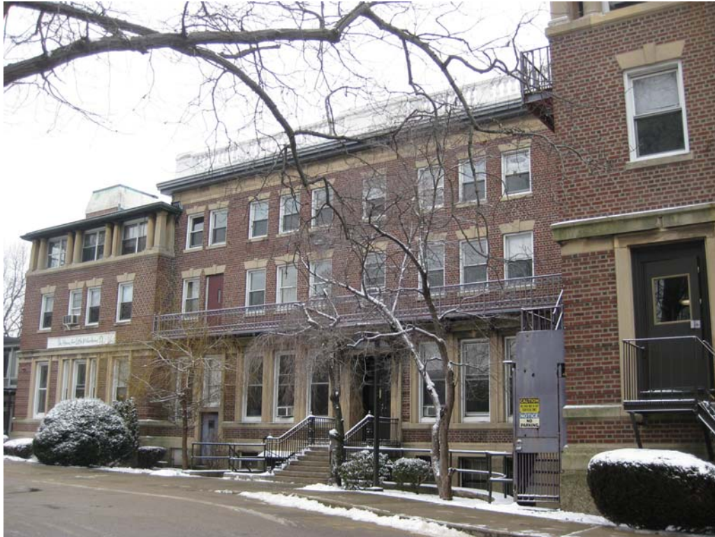
3. Home for Little Wanderers, 1914 Building (east elevation)
