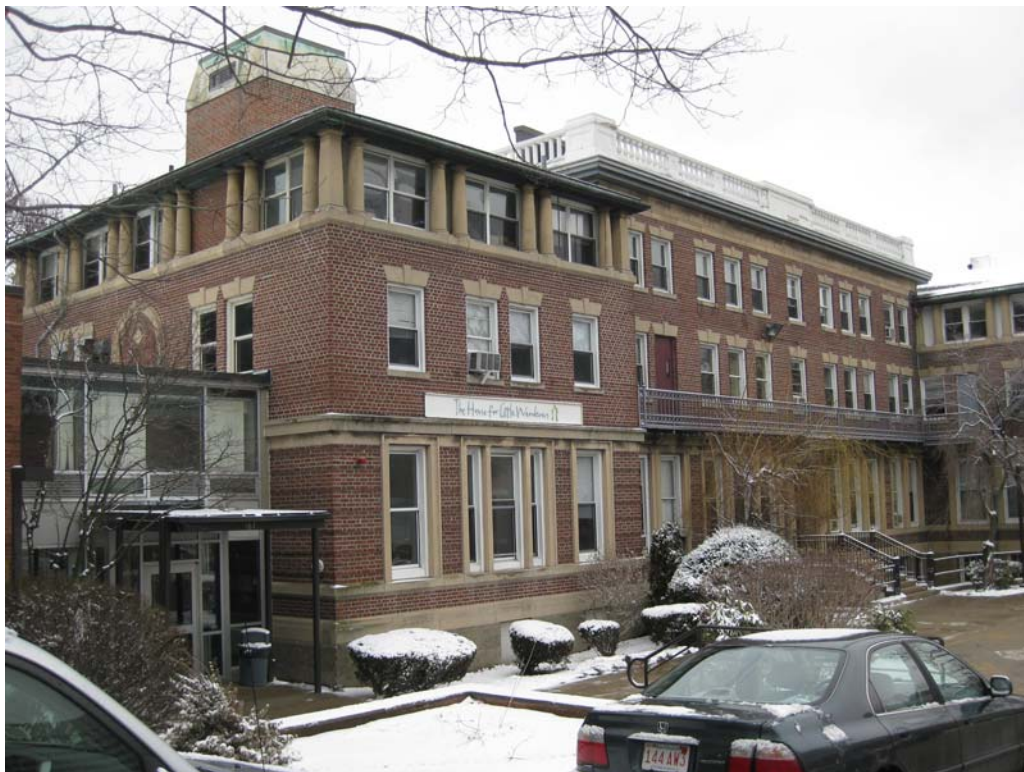
4. Home for Little Wanderers, 1914 Building (south and east elevations)
