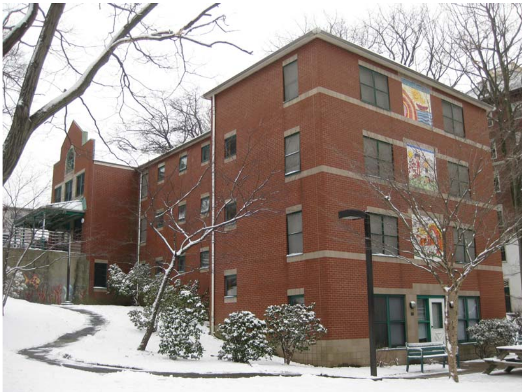
10. 1987 Residential Building (north and west elevations)
