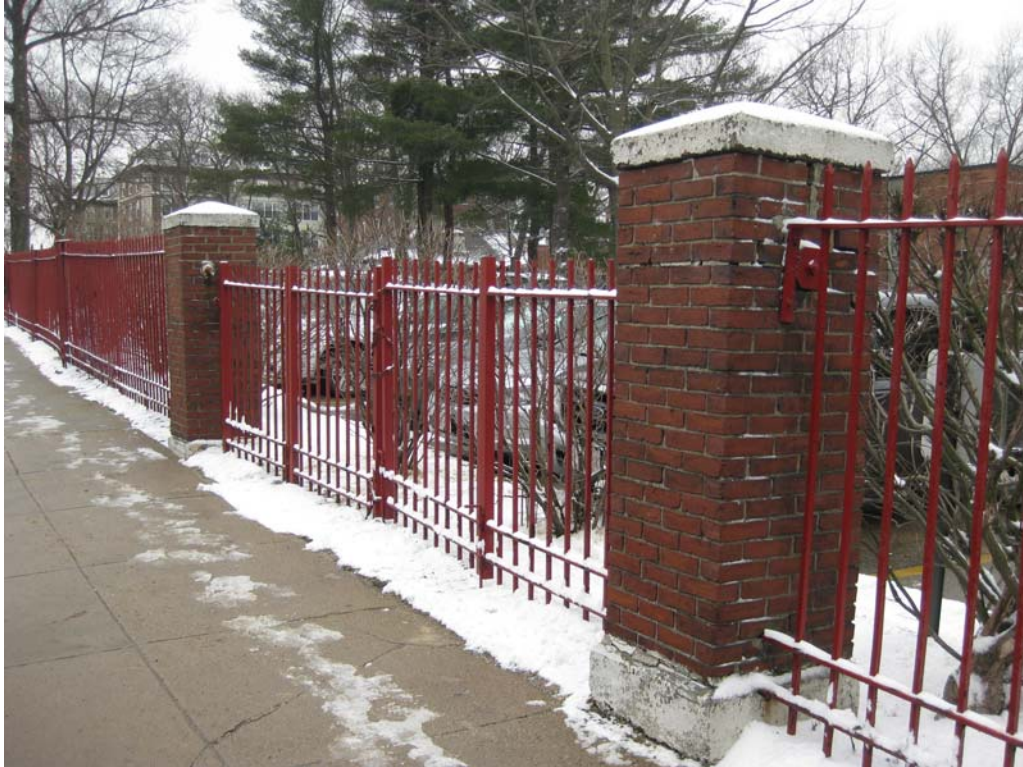
13. Iron picket fence on South Huntington Avenue
