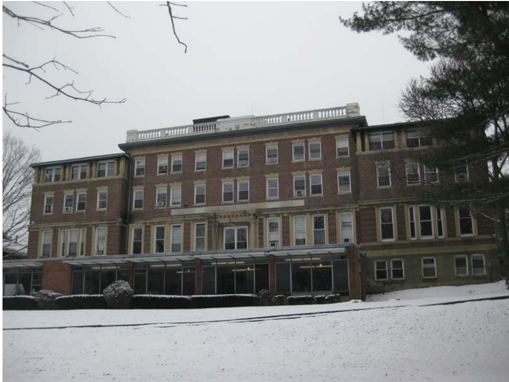
7 1914 Building and 1950s addition (west elevation)
