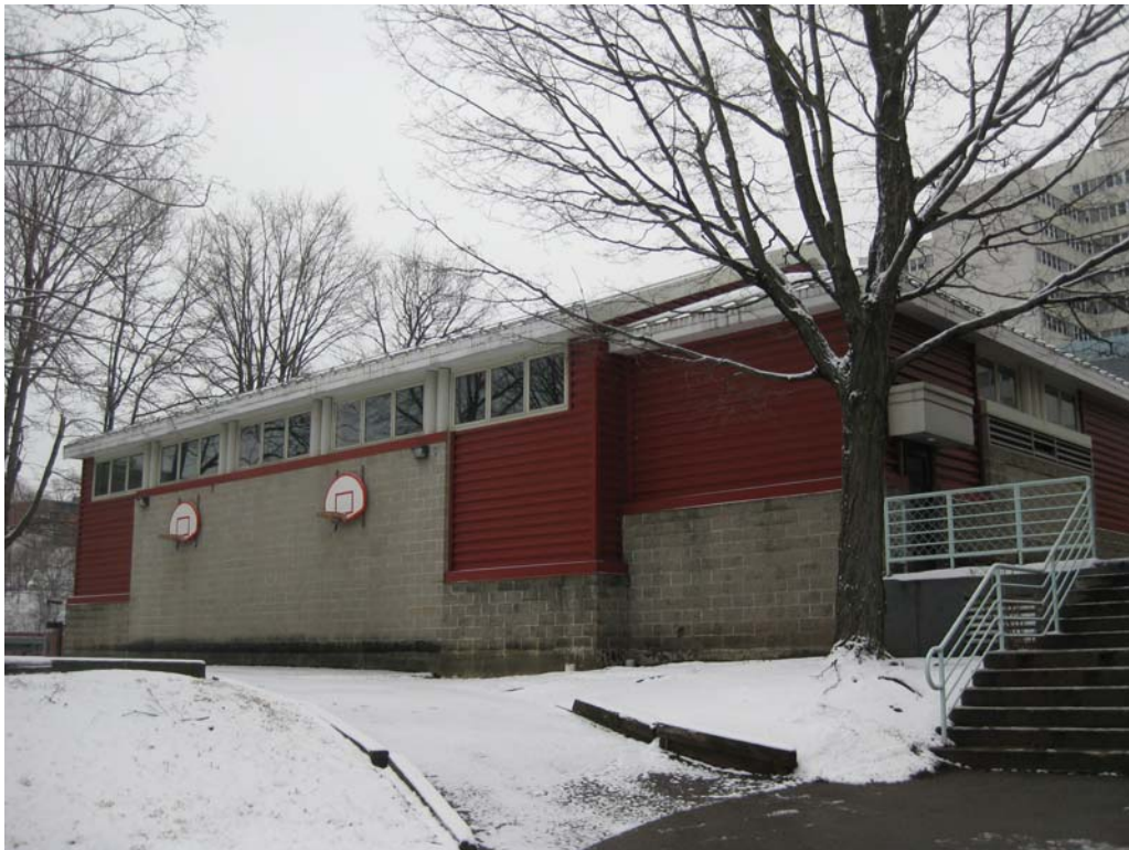
12. 1991 Gymnasium (west and south elevations)
