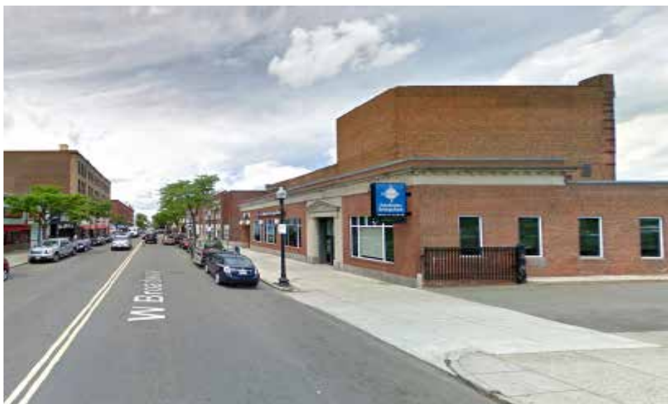
3. EAST FACADE FROM WEST BROADWAY
