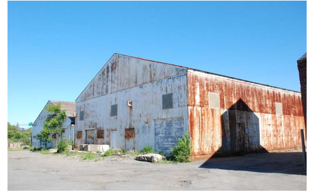
Existing Boat Storage
