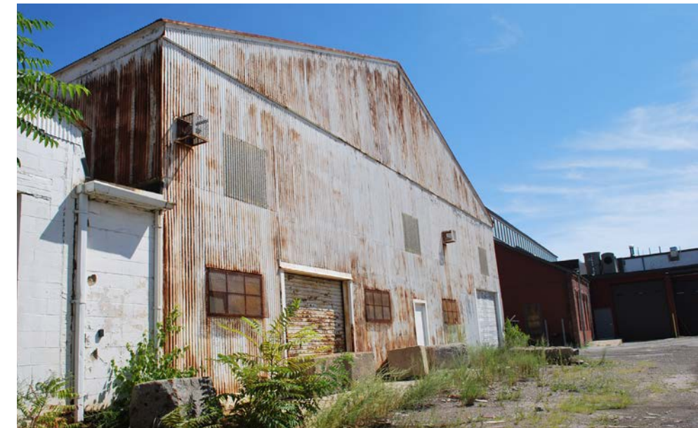
Existing Boat Storage
