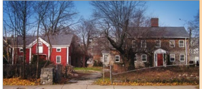
The Fowler Clark Epstein Farm before rehabilitation.
