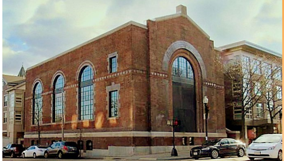
Roslindale Substation Exterior Restoration Fall 2016
