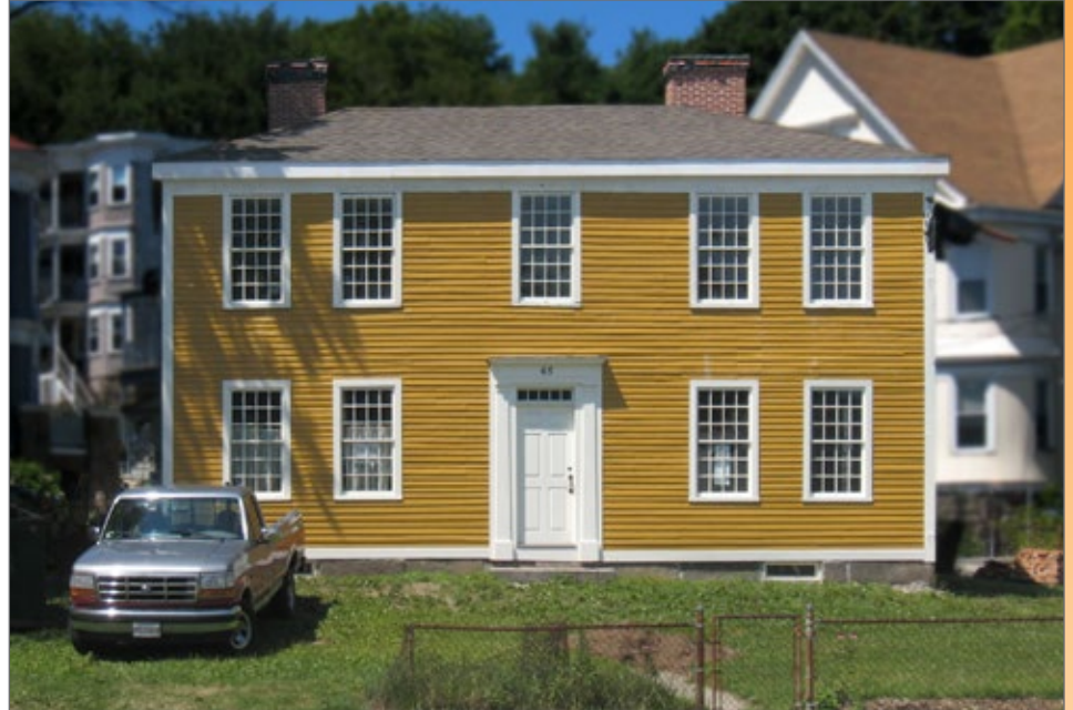
HBI and North Bennet Street School were partners on the preservation of the 1804 Anna Clapp Harris Smith house.
