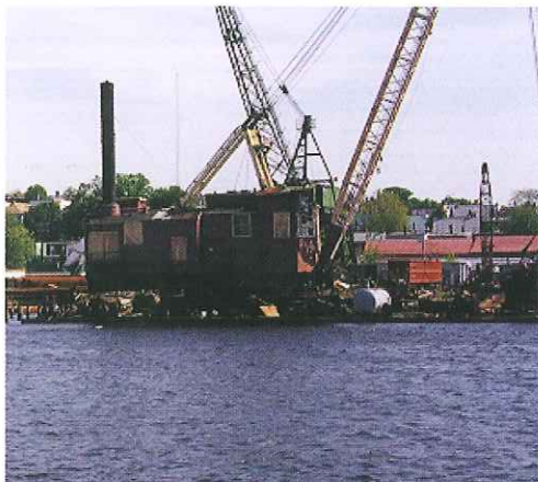
Existing industrial waterfront
