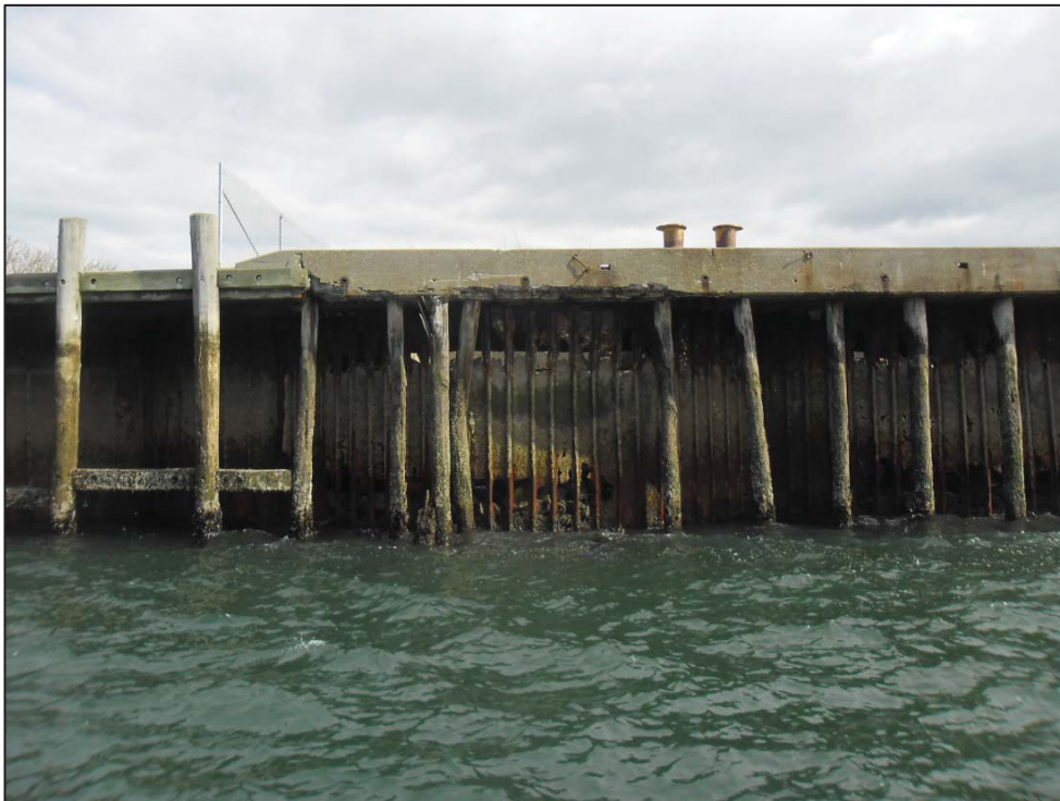
Figure 20: View of perforated steel bulkhead along Dry Dock #4.
