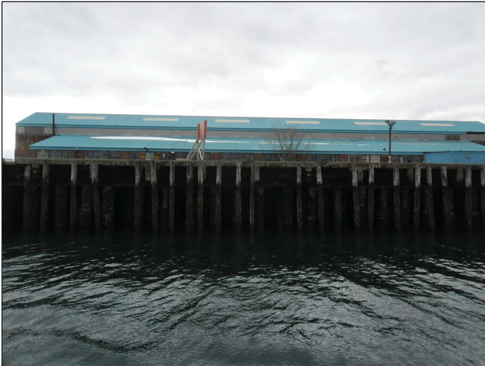
Figure 11: View of pile encasements along the East Jetty.
