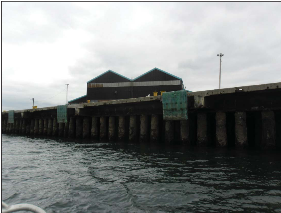
Figure 13: Overall view of the existing North Jetty wharf and fender system.
