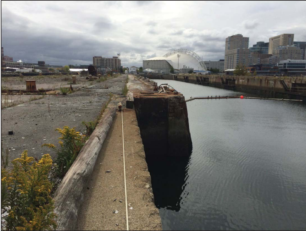
Figure 17: Dry Dock #4 berth, looking south.
