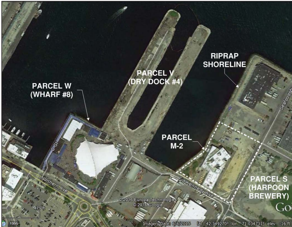
Figure 15: Aerial view of BMIP Parcels V and W.
