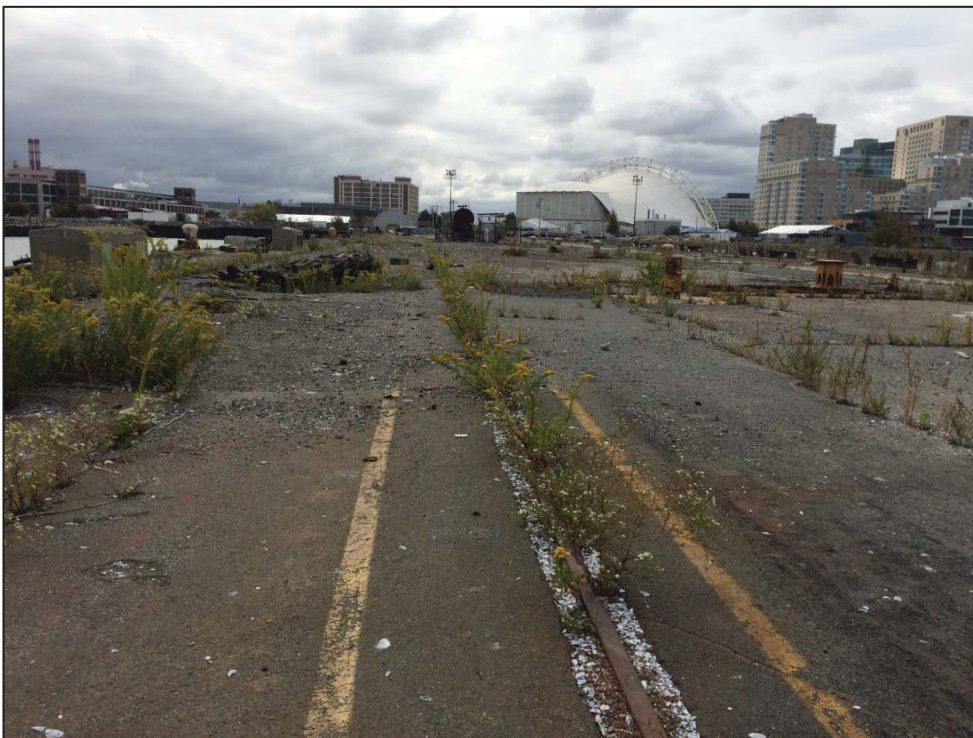
Figure 18: Overall view of the deck at Dry Dock #4.
