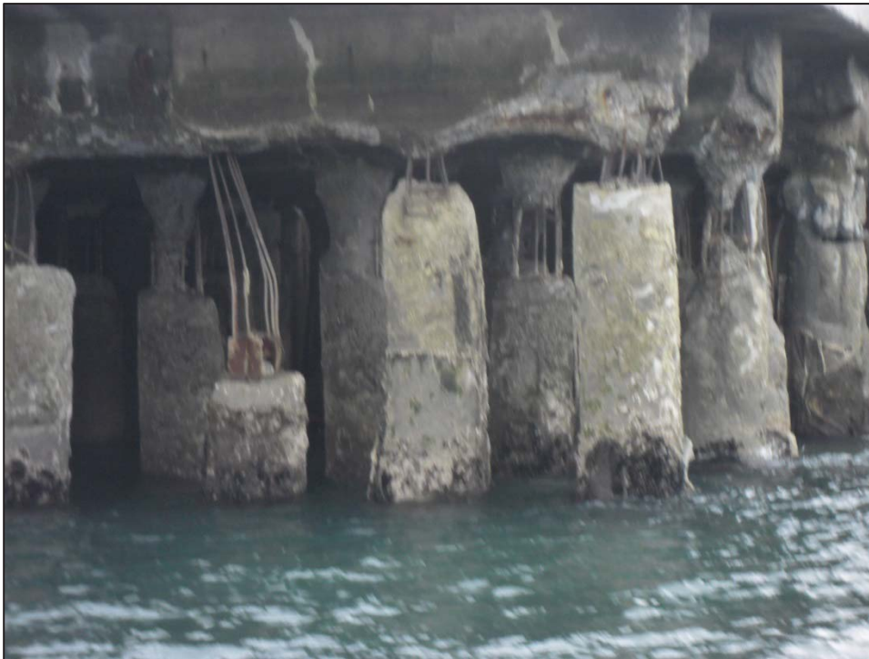
Figure 14: Typical condition of piles supporting the North Jetty wharf deck.
