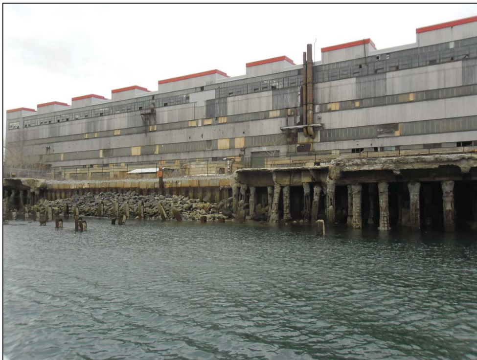
Figure 10: Existing conditions at South Jetty.
