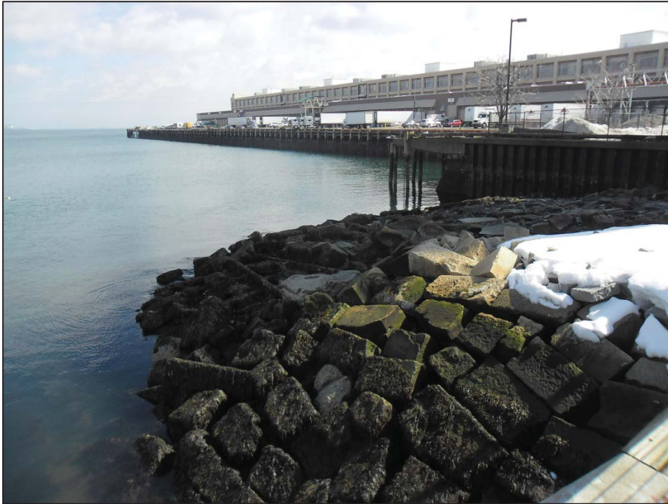
Figure 22: Overall view of Pier 10 and Massport Berths 1 and 2 (in background).
