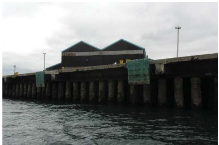
Parcel M viewed from the North Jetty
