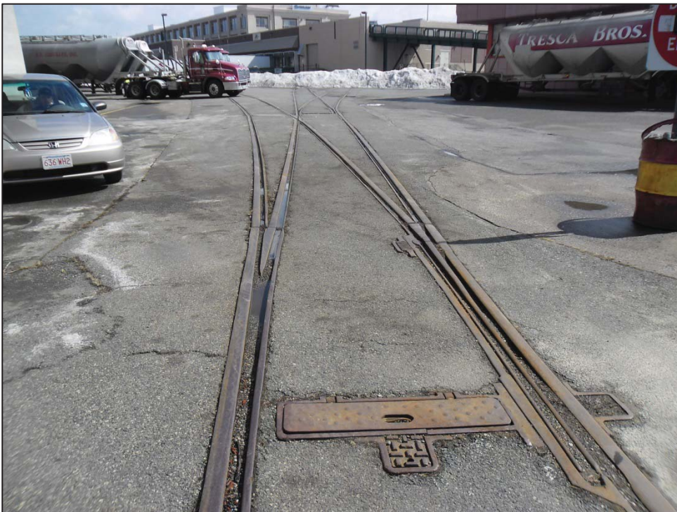
Figure 5: View of Track 61 rail infrastructure at Parcel K in the east end of the BMIP.
