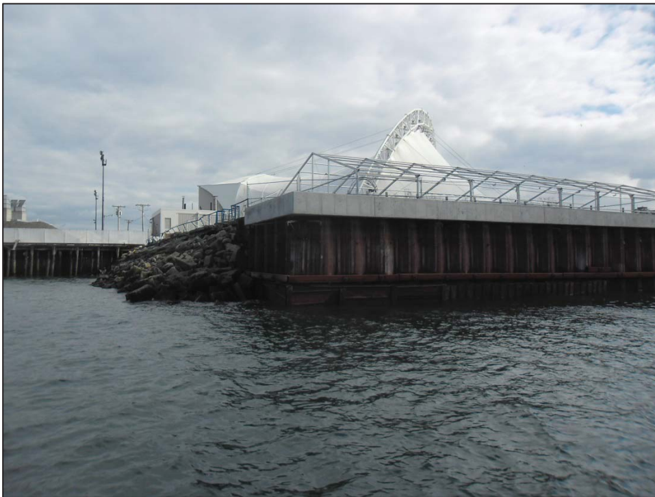
Figure 21: Overall view of recent steel bulkhead and riprap repairs at Wharf 8.
