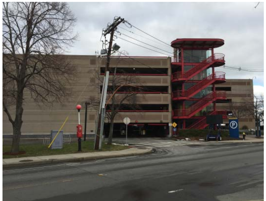
The EDIC parking deck (Parcel Y) is the only dedicated parking structure in the RLFMP.
