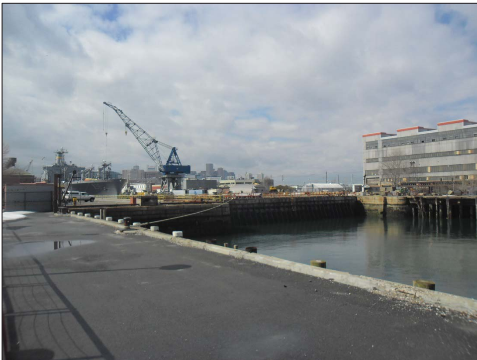
Figure 23: View of the deck at Pier 10, looking east towards Dry Dock #3.
