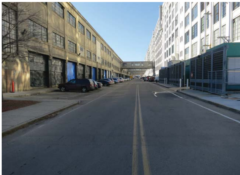
Black Falcon Ave provides rear loading access for 27 Drydock, the IDB and the Massport Cruise Terminal.
