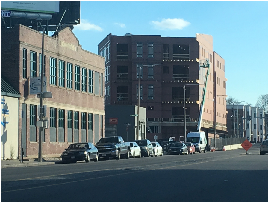
View of New Construction Next to 200-204 Old Colony Ave
