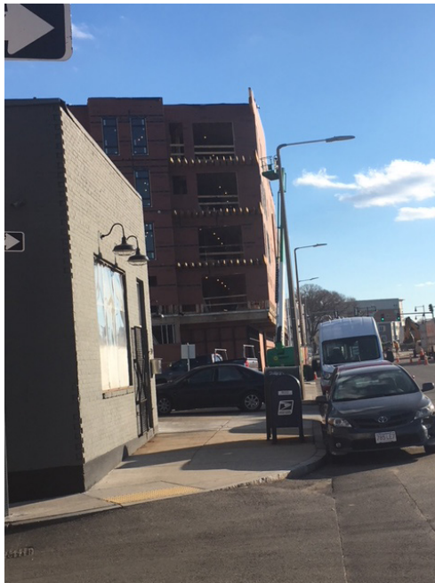
Adjacent New Construction Along Old Colony Ave
