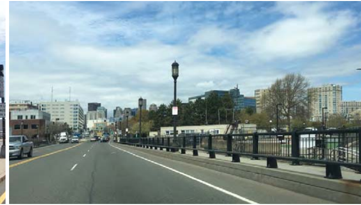
_SUMMER STREET BRIDGE
