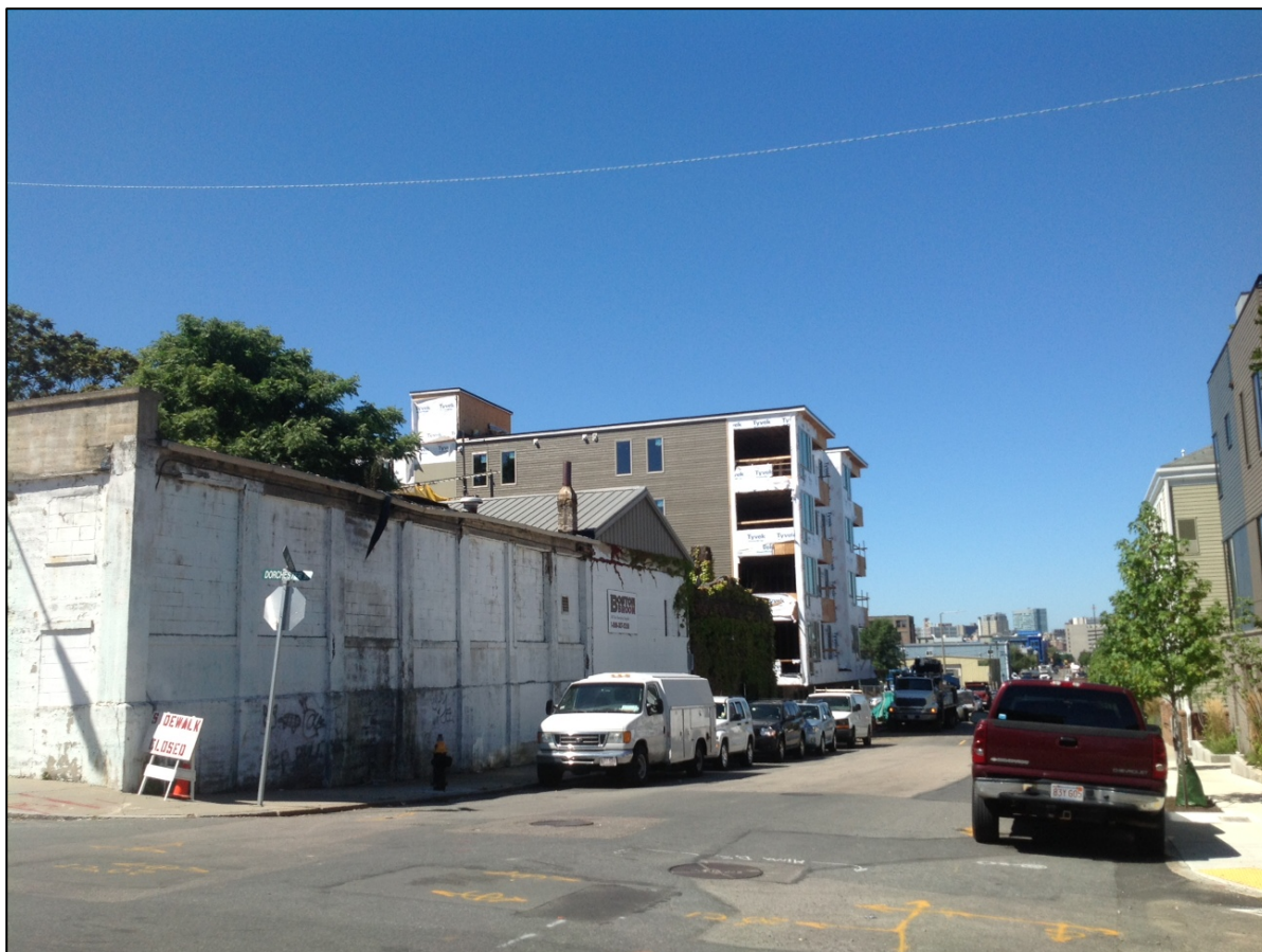
EXHIBIT 4 - VIEW DOWN WEST FIRST STREET
