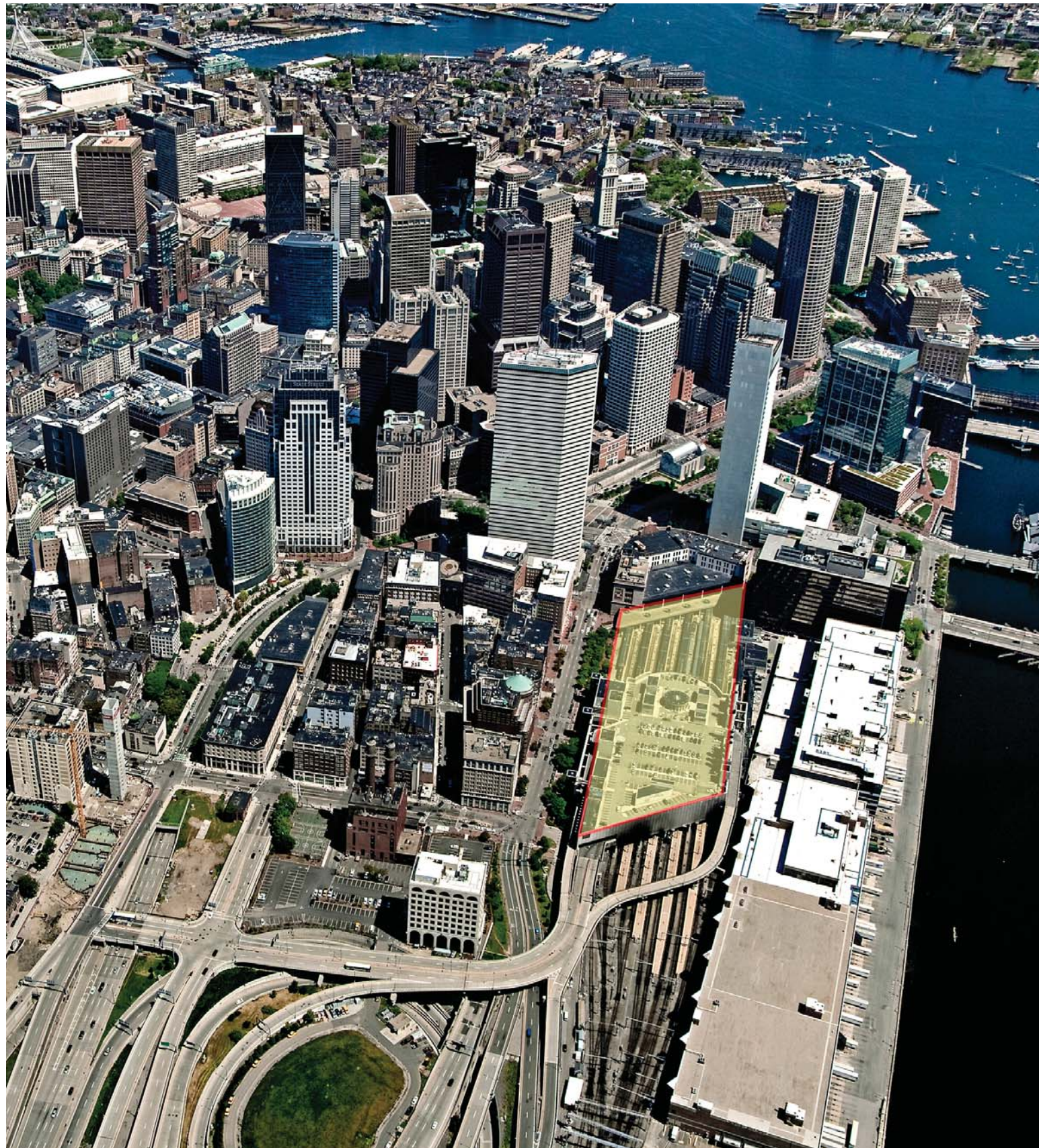
EXISTING CONDITIONS - AERIAL PHOTO
