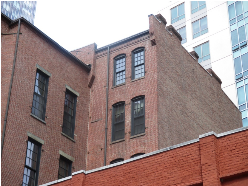
23. Rear (south) and side (west) elevations of 1883 addition
