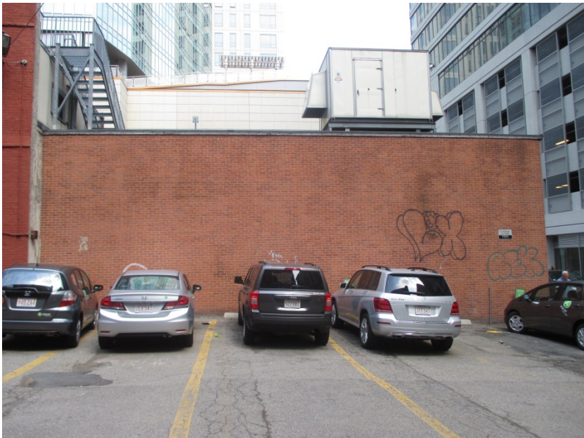
27. Side (west) elevation of 1956 addition
