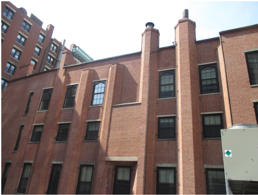
21. Rear (south) elevation of 1875 building
