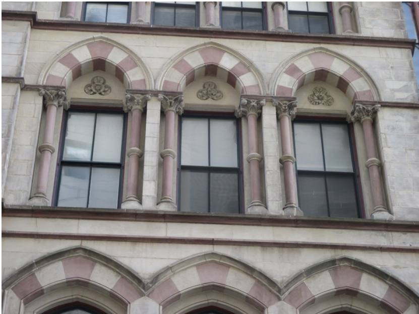
7. Front (north) elevation, second floor window detail
