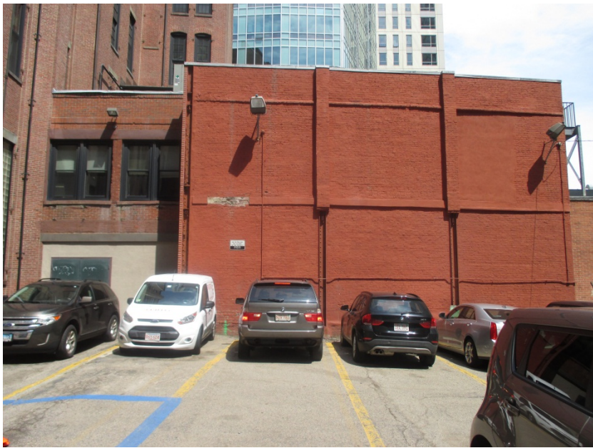
25. Side (west) elevation of 1911 addition
