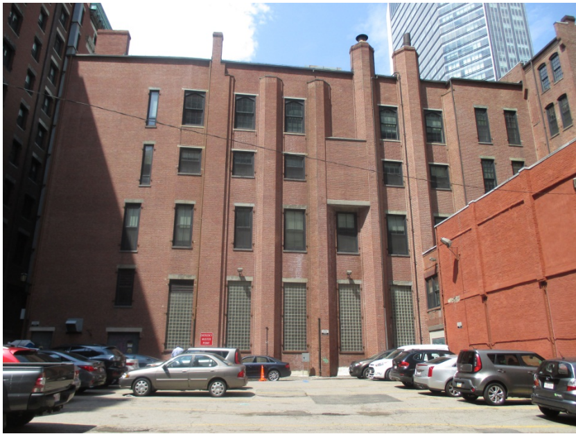
17. Rear (south) elevation of 1875 building
