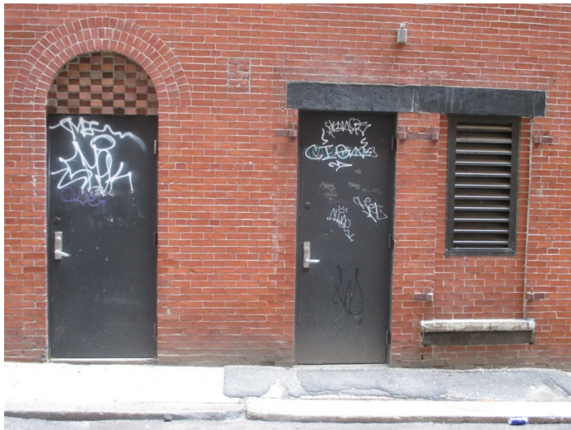
13. Side (west) elevation, basement entrances and infilled window
