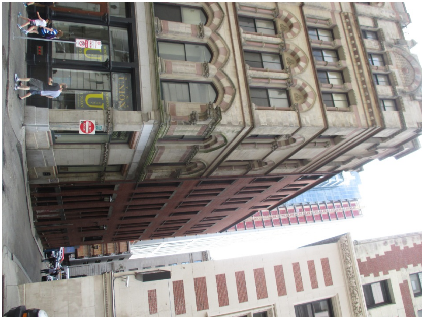
9. Side (west) and front (north) elevations
