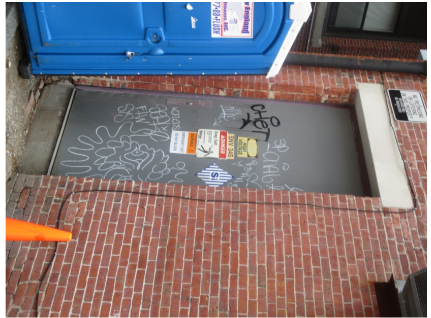
18. Rear (south) elevation, entrance detail
