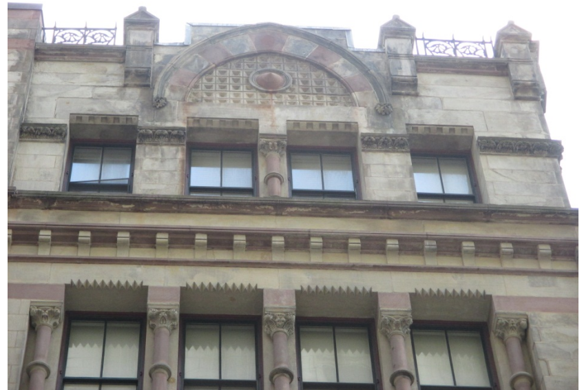
8. Front (north) elevation, fourth and fifth floor window and masonry detail
