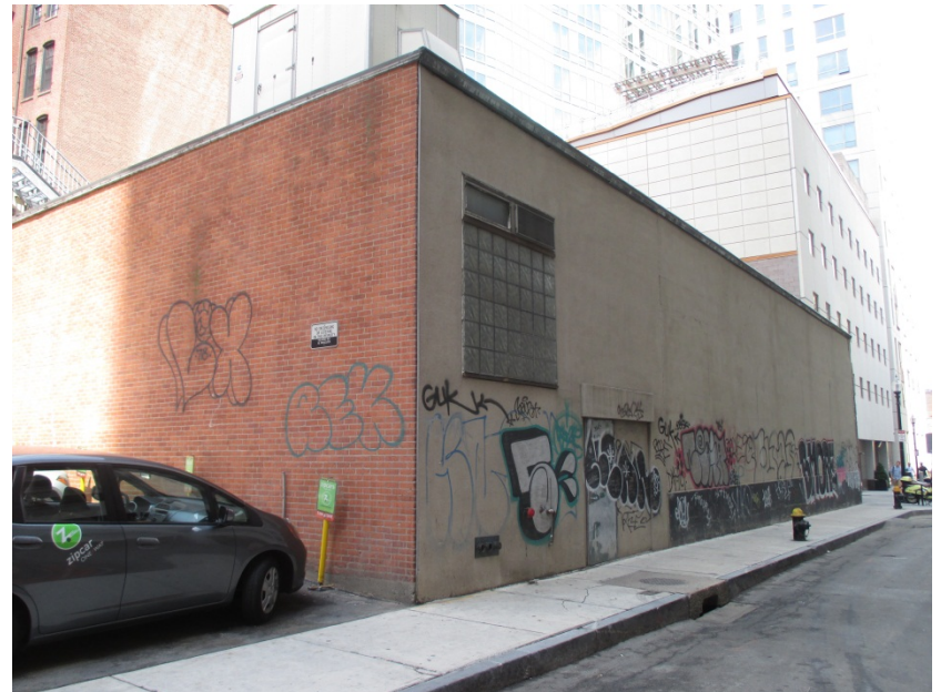
28. Side (west) and rear (south) elevations of 1956 addition
