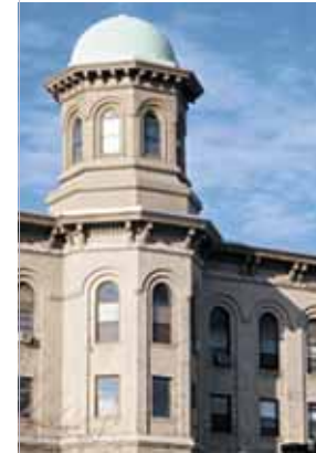
The Piano Factory is a creative, adaptive reuse of a former industrial building for housing
