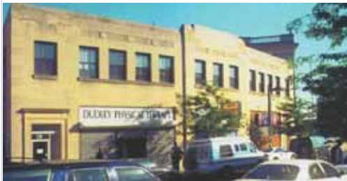
Before view of Roxbury storefront
