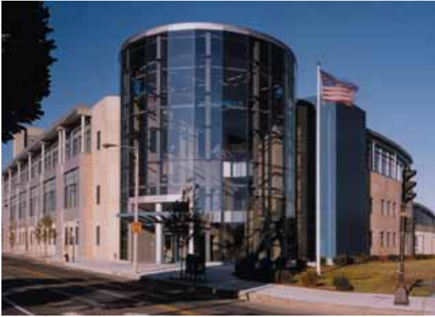
Boston Water and Sewer Commission's new headquarters
