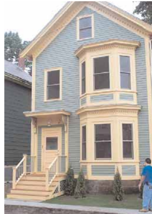
Recently completed housing on Stanwood Street
