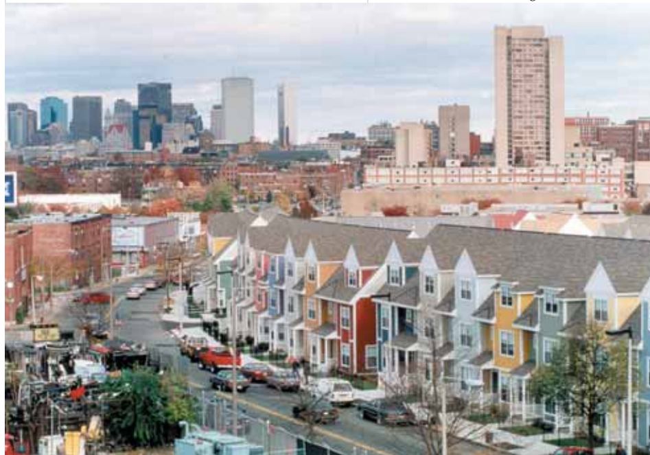
New housing at Orchard Gardens
