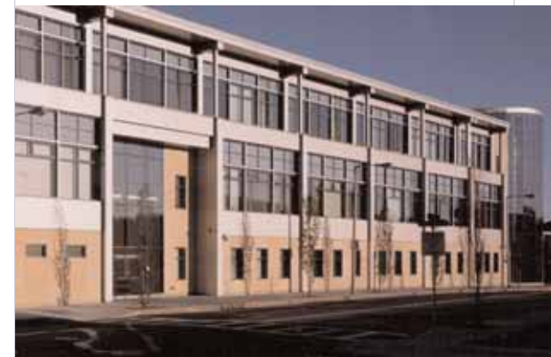
Boston Water and Sewer Commission headquarters
